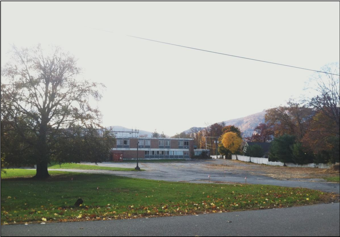
View 1 from Paulding Avenue, looking SW.
