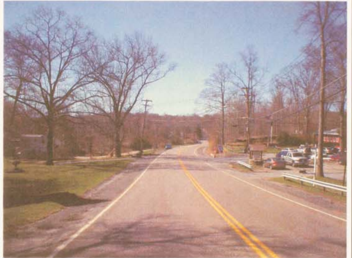
2) Oscawana Lake Road 900-1300 feet north of Town Hall
