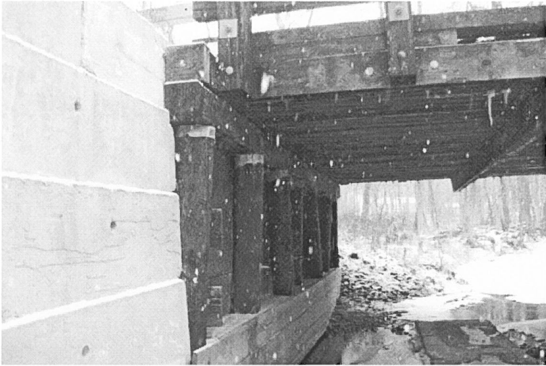
Photo 13: East Abutment looking South
