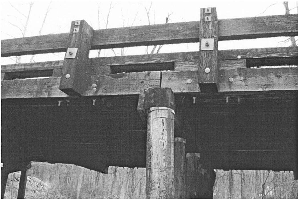
Photo 4: End of Pier
