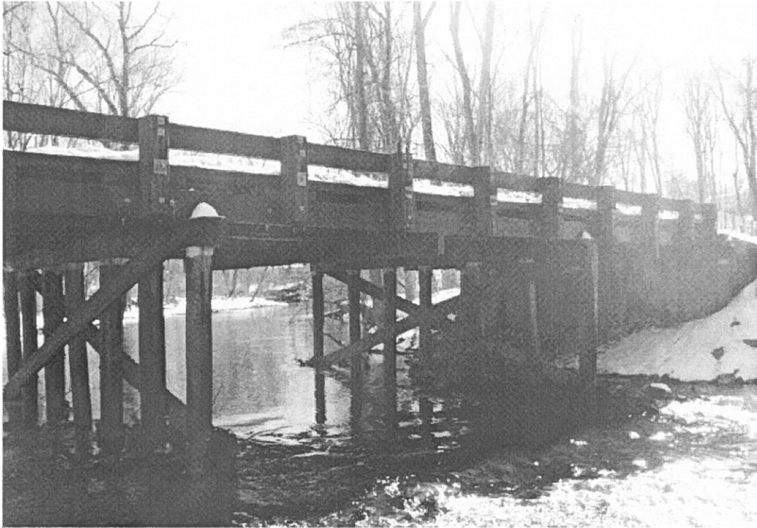
Photo 3: Bridge Elevation looking South
