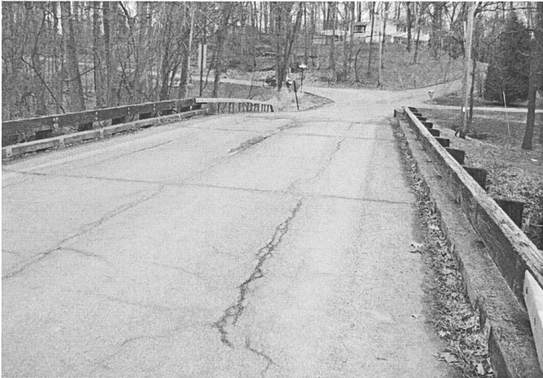
Photo 1: On Bridge looking West
