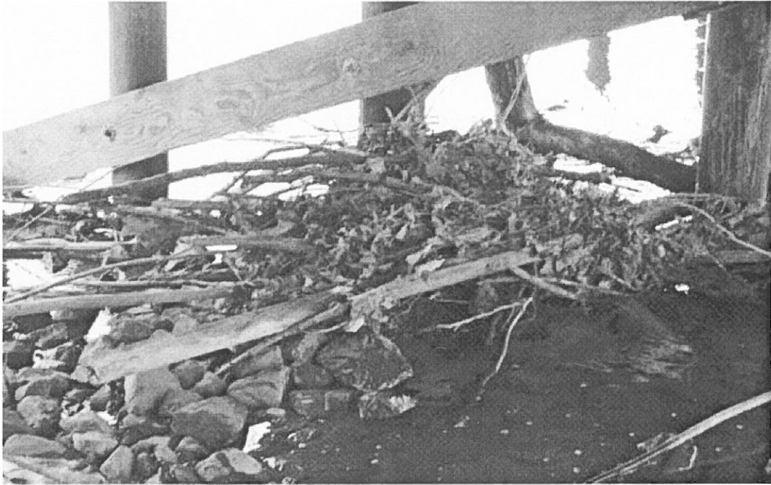
Photo 10: Debris in steam under bridge between West Abutment and Pier 1
