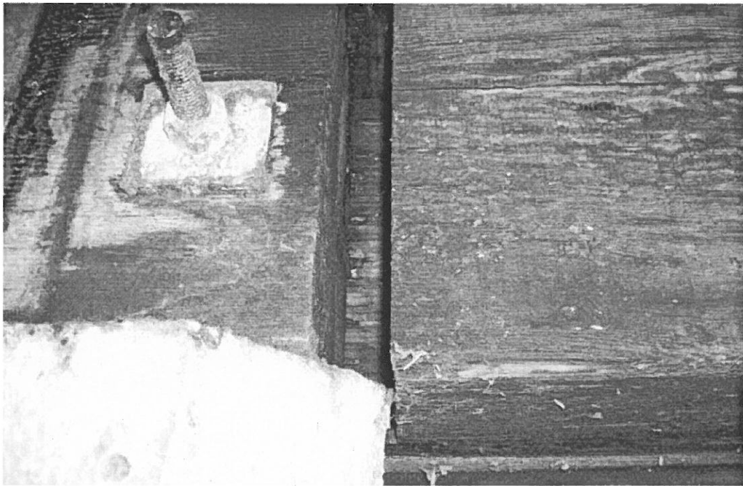
Photo 8: West Abutment Cap Beam Splice off Pile
