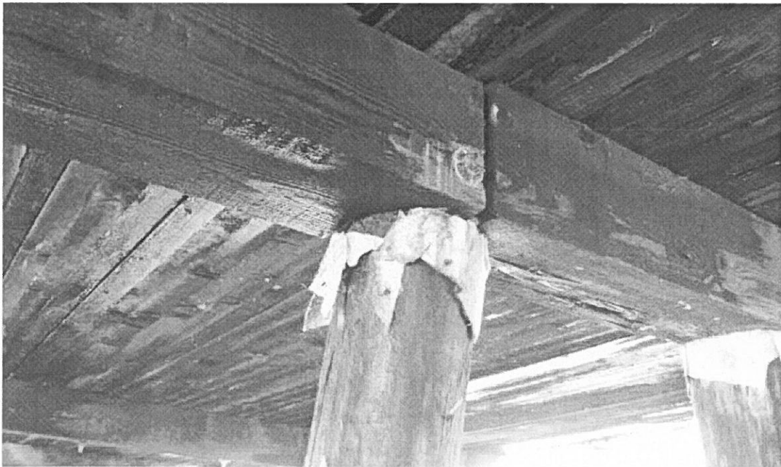
Photo 6: Pier 1 Cap Beam Splice
