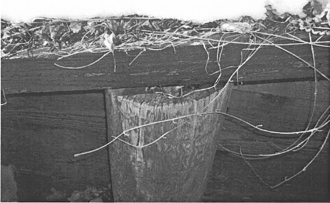
Photo 5: SW Wingwall Pile with rot at top
