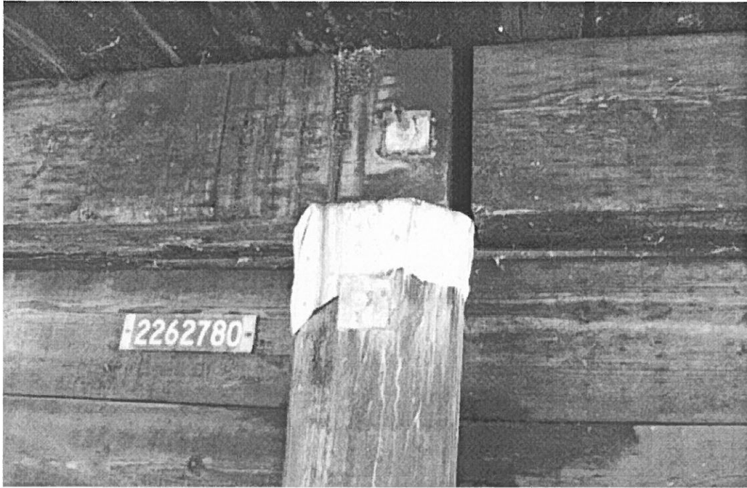
Photo 11: West Abutment Cap Beam Splice off Pile
