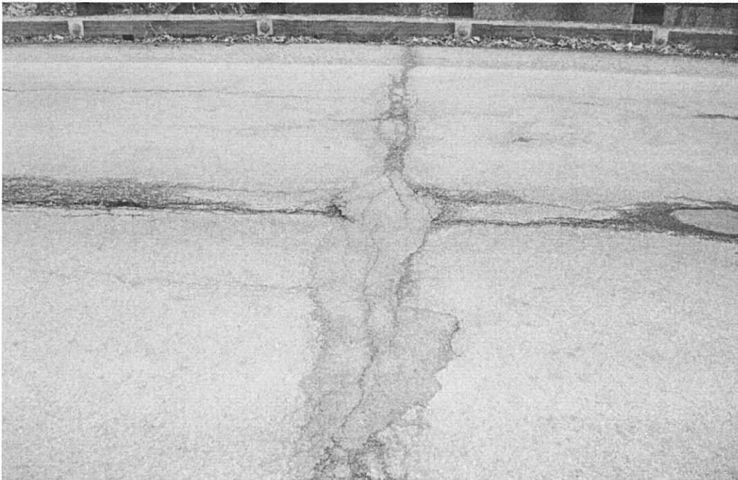
Photo 2: Crack in Asphalt at Pier
