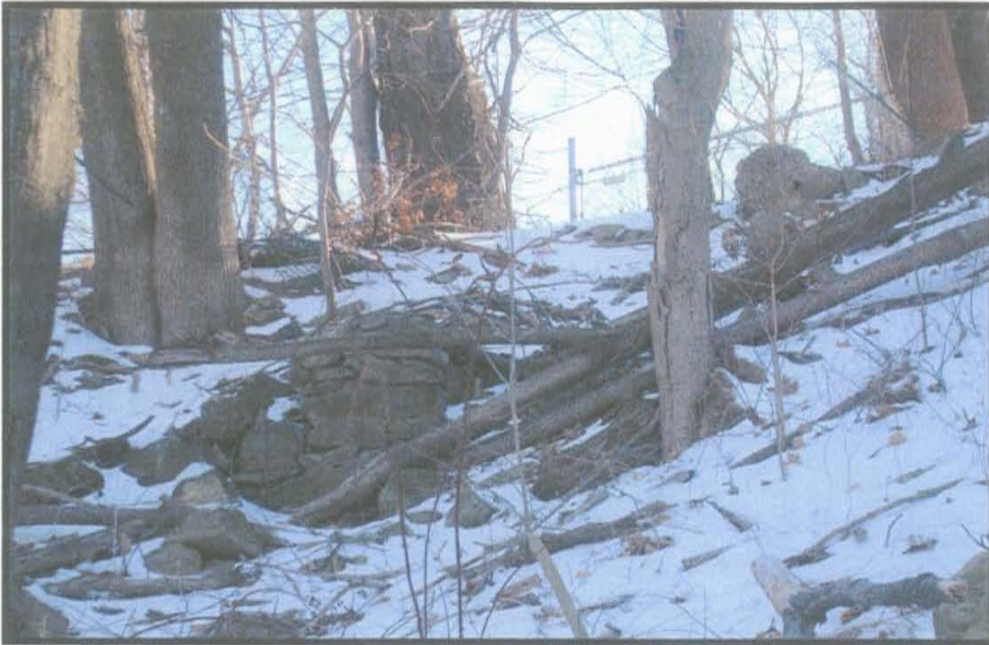
Photo 13: Small fieldstone construction, possibly part of a foundation, located in south central portion of site. View to south, with fence lining Pipe Town Hill in background.
