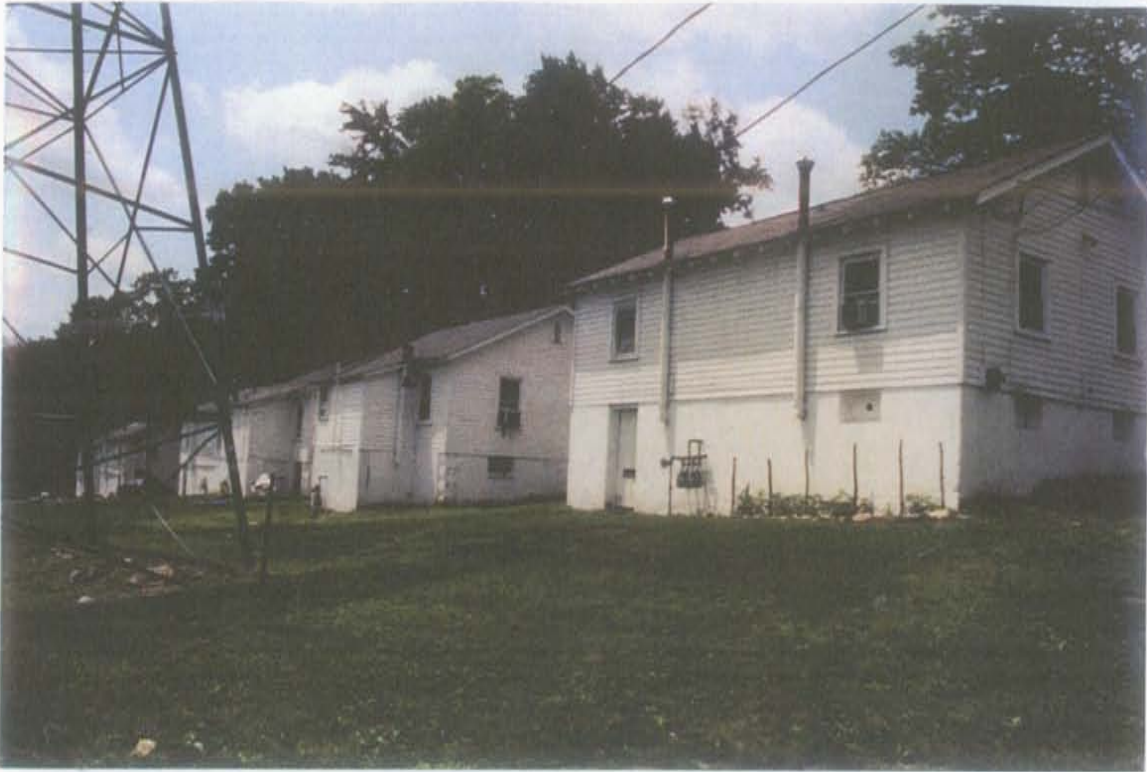
PHOTO 3 - Line of existing bungalows in east-central area (view to SSW)
