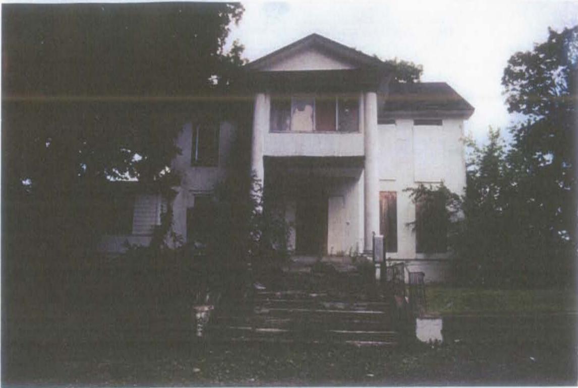
PHOTO 1 - Potentially Eligible Structure (PES) (view to W)
