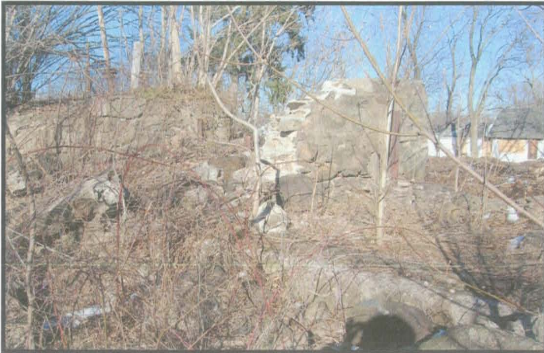
Photo 10: Close up view of stone and mortar remains, with concrete and iron features. On-site dwellings in background. View to northeast.
