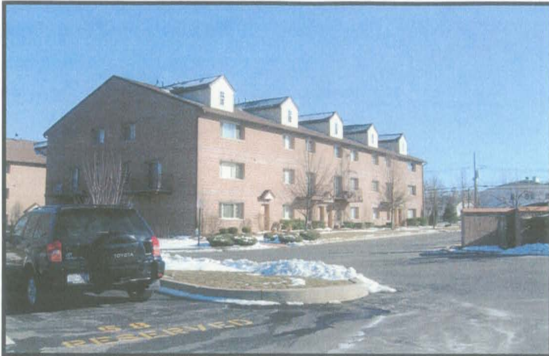
Photo 1: The Conklin Park Condominium's parking lot. Pipe Town Hill Road in background. View to south.
