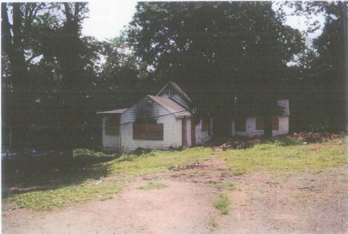
PHOTO 6 - Fire-damaged structure in southeast corner of complex (view to S)
