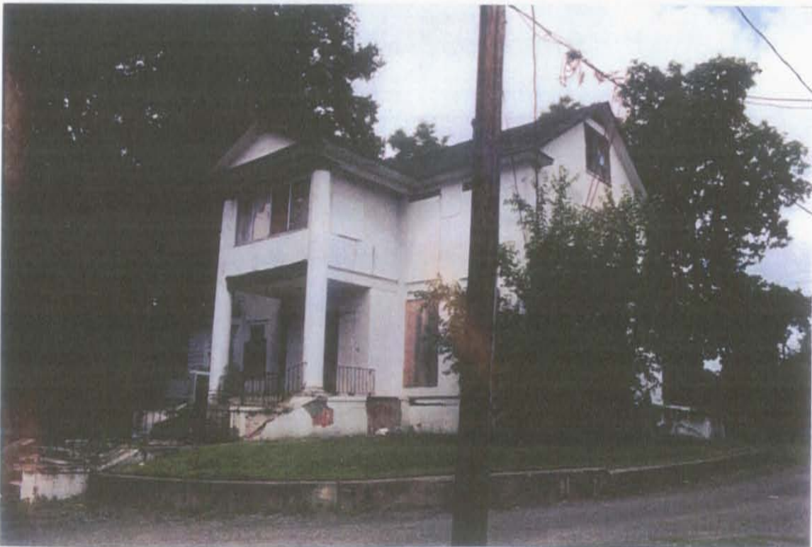
PHOTO 2 - Potentially Eligible Structure (view to SW)
