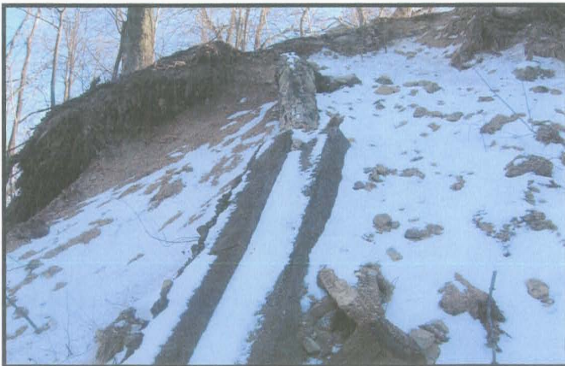
Photo 12: Concrete construction materials, likely associated with former dam and roadway. View to south, looking up towards location of concrete foundation.
