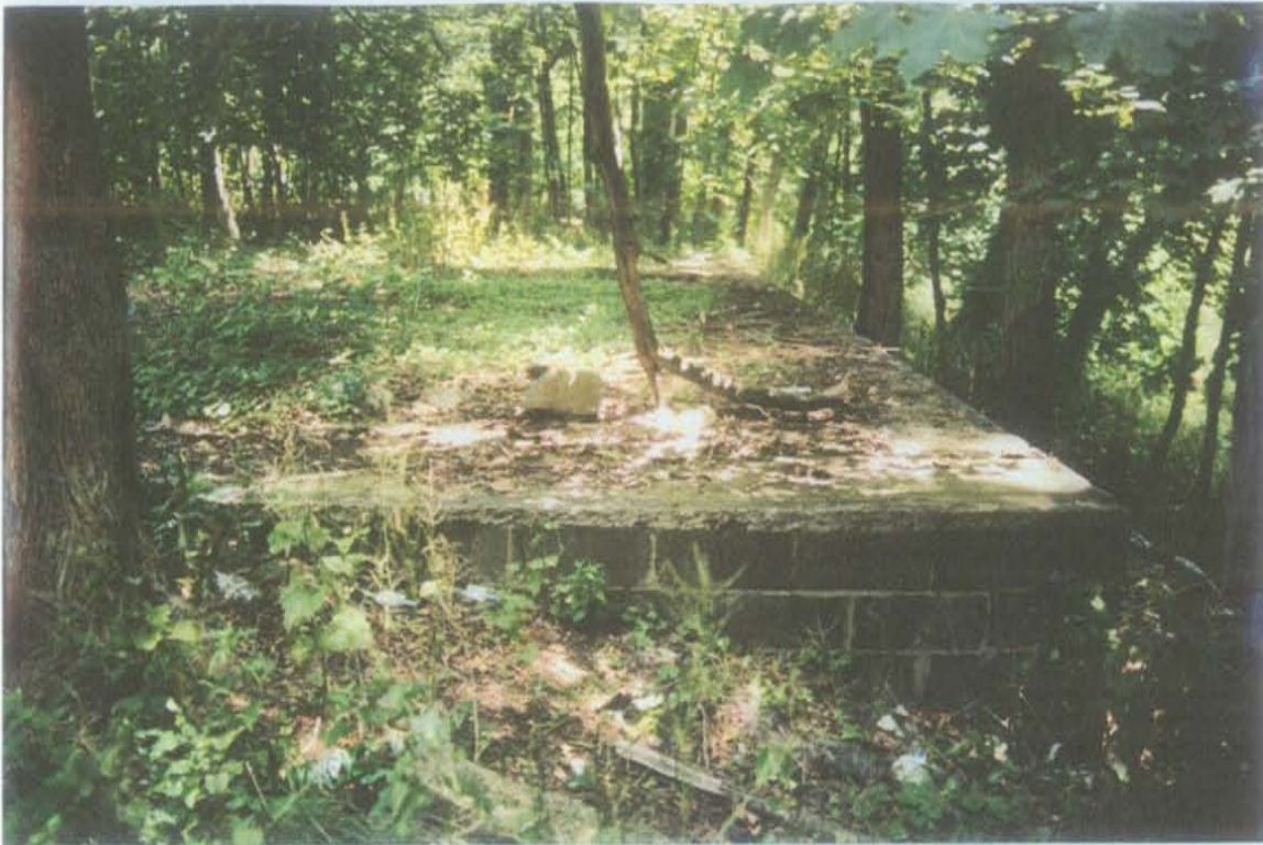
PHOTO 9 - Concrete block recreational structure in west-central area (view to W)
