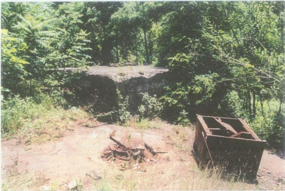
PHOTO 10 - Concrete support structure in western part of parcel (view to SW)
