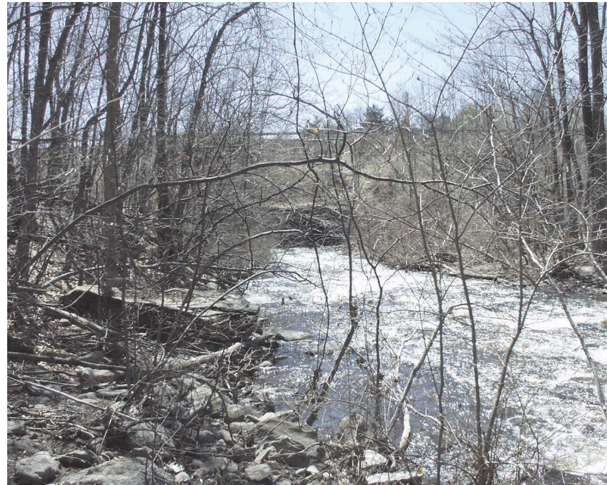
C: Box culvert under I-84 located off-site.
