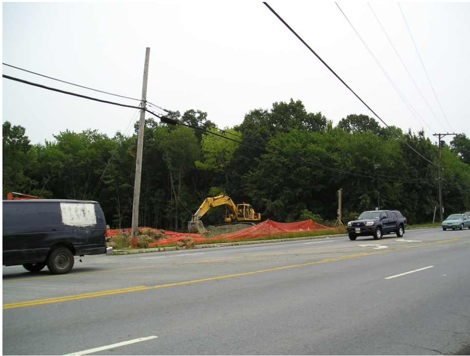
View Towards Project Site from Route 300
