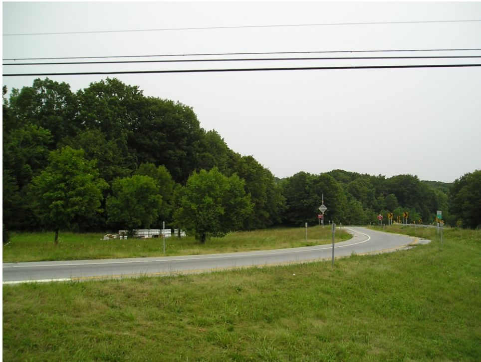
View Towards the Project Site from Route 300 - Route 84 Ramp
