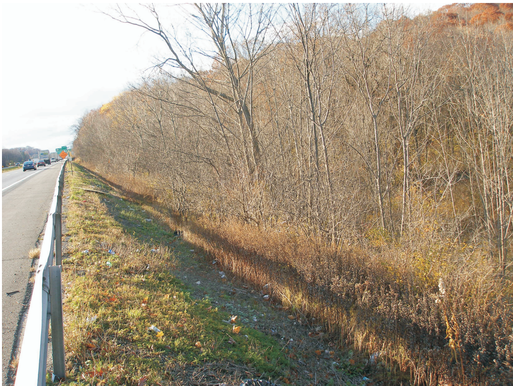
View from I-84 looking West
