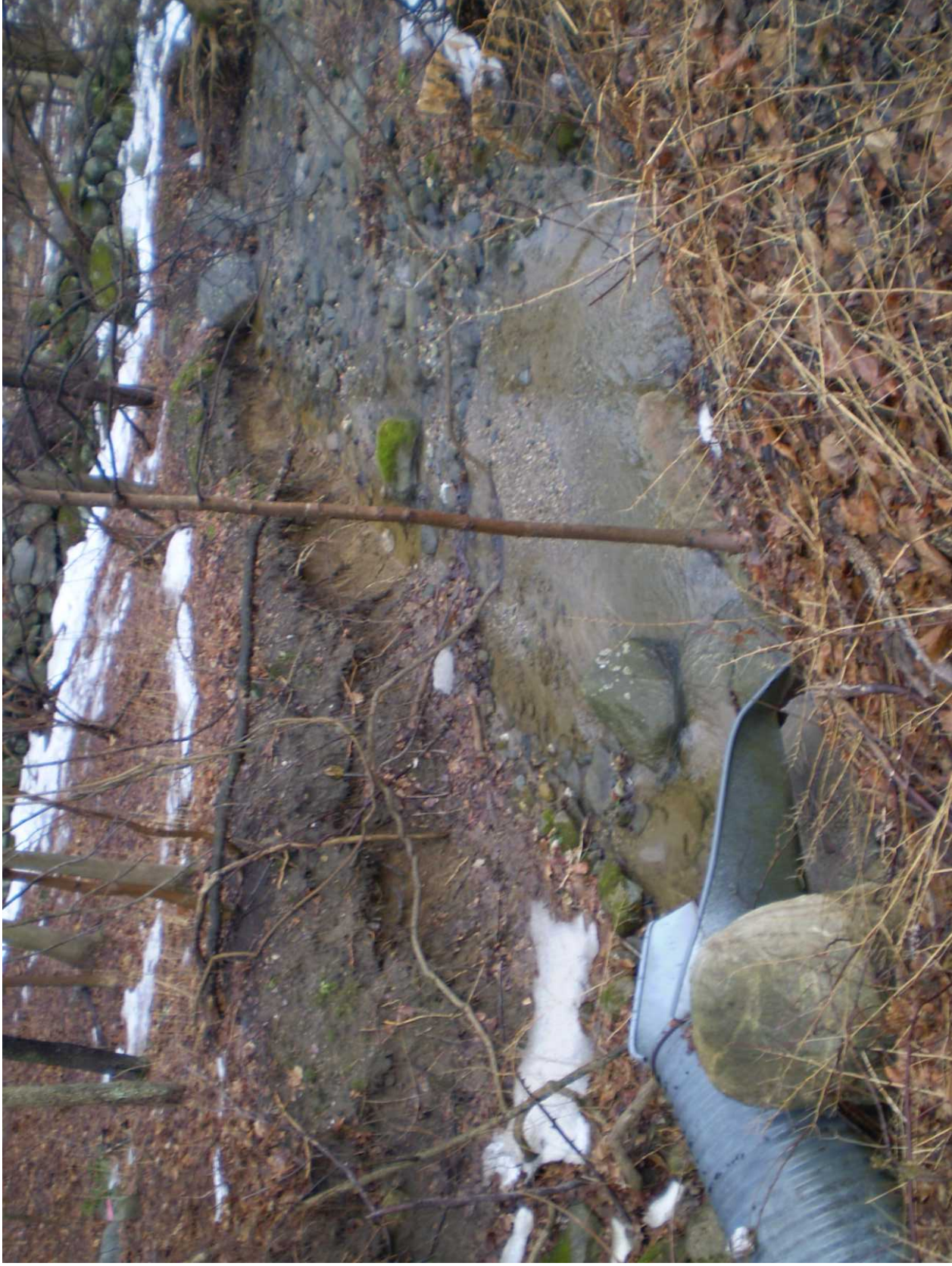
Figure 4.5-6: Eroding Drainage Channel - Along NYS Route 311 Patterson Crossing Town of Patterson, Putnam County, New York Source: TMA Photograph, 01/09/08
