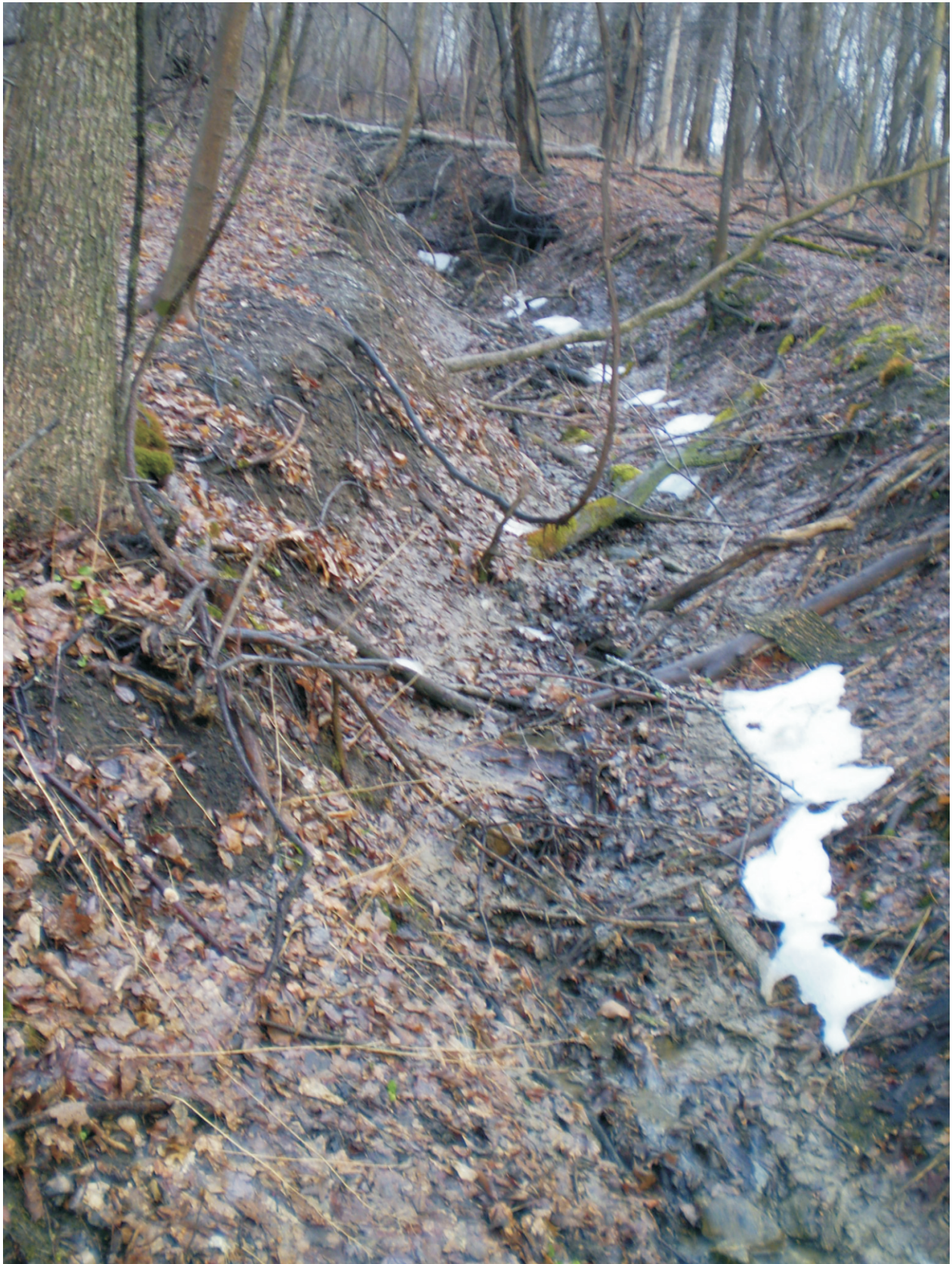
Figure 4.5-5: Eroding Drainage Channel From Concord Road Patterson Crossing Town of Patterson, Putnam County, New York Source: TMA Photograph, 01/09/08
