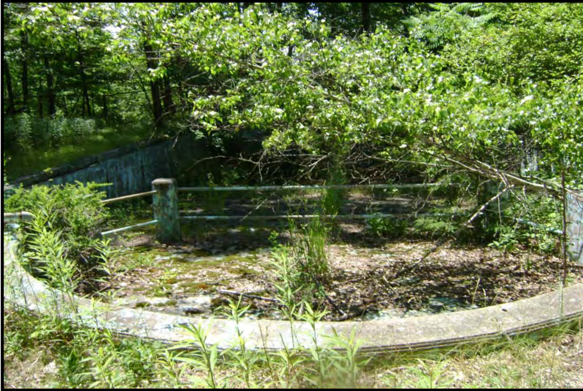
Photo 23: Swimming pool located in northeastern corner of Raleigh Hotel Site View west.
