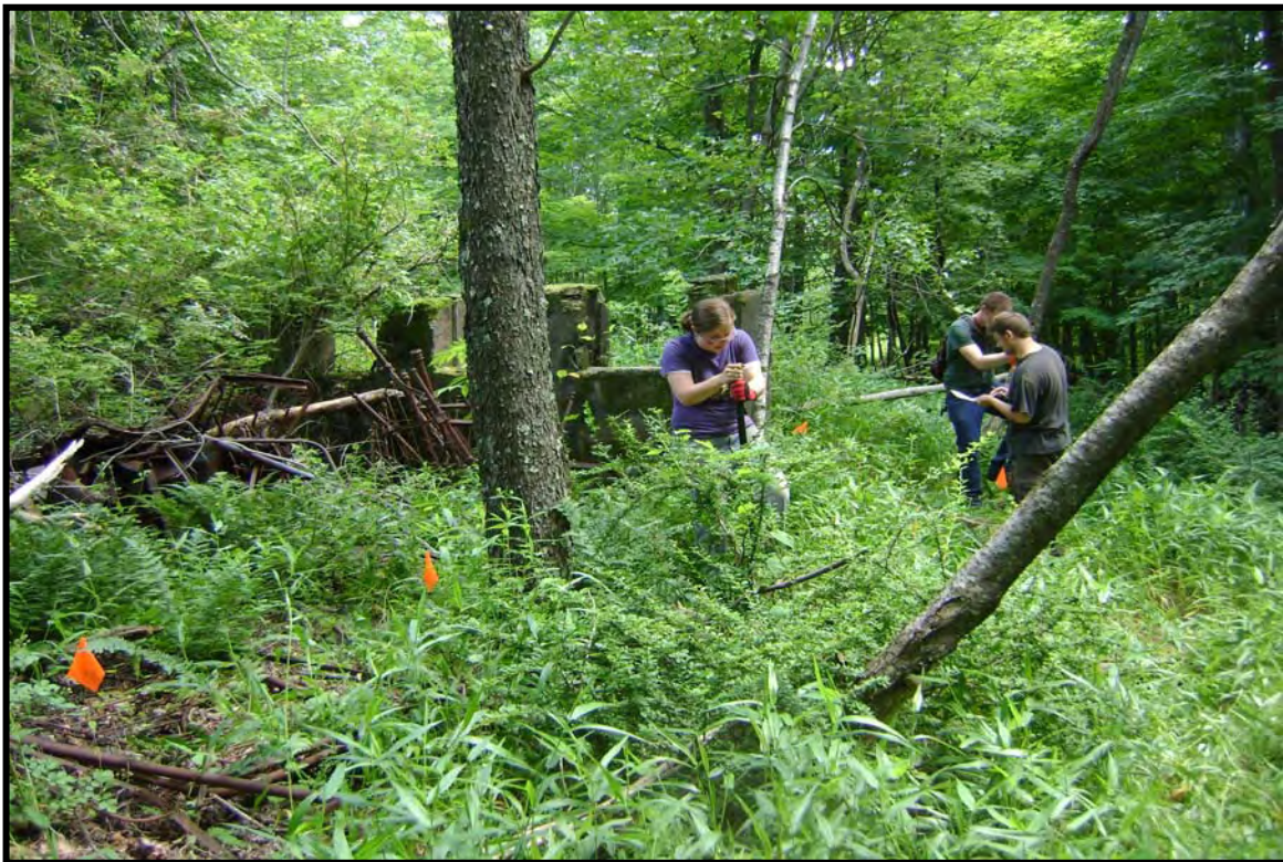
Photo 28: Stone and concrete foundation identified on eastern boundary of the APE, near Fred Road. Perimeter tested at 5' interval. View northeast.
