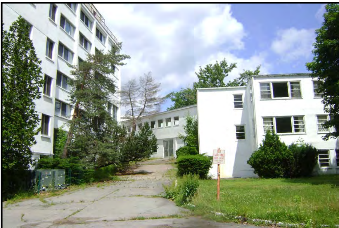
Photo 18: Existing and operational Raleigh Hotel. View northwest.
