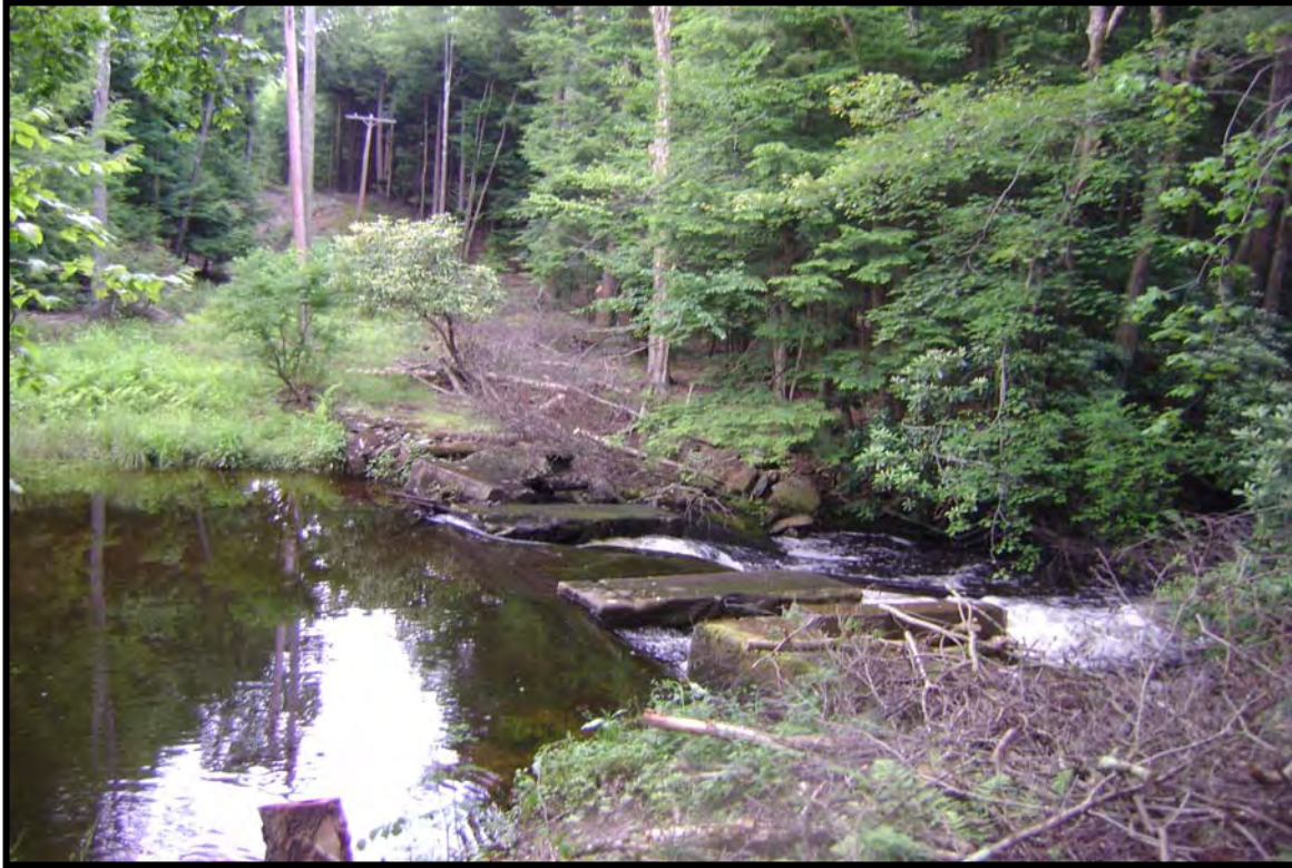
Photo 9: Concrete spillway and bridge over Sheldrake Creek. View east.
