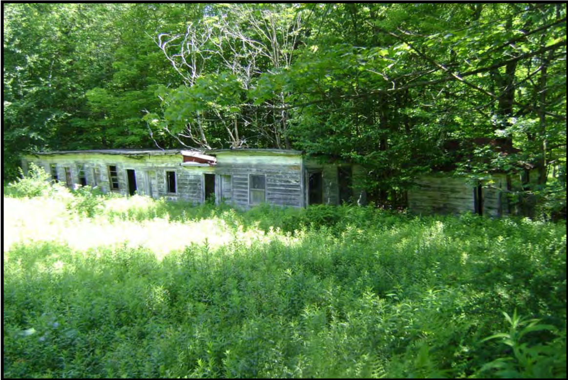
Photo 4: Unidentified structure located in rear of former Heiden Hotel parcel. Structure has no foundation. View northeast.
