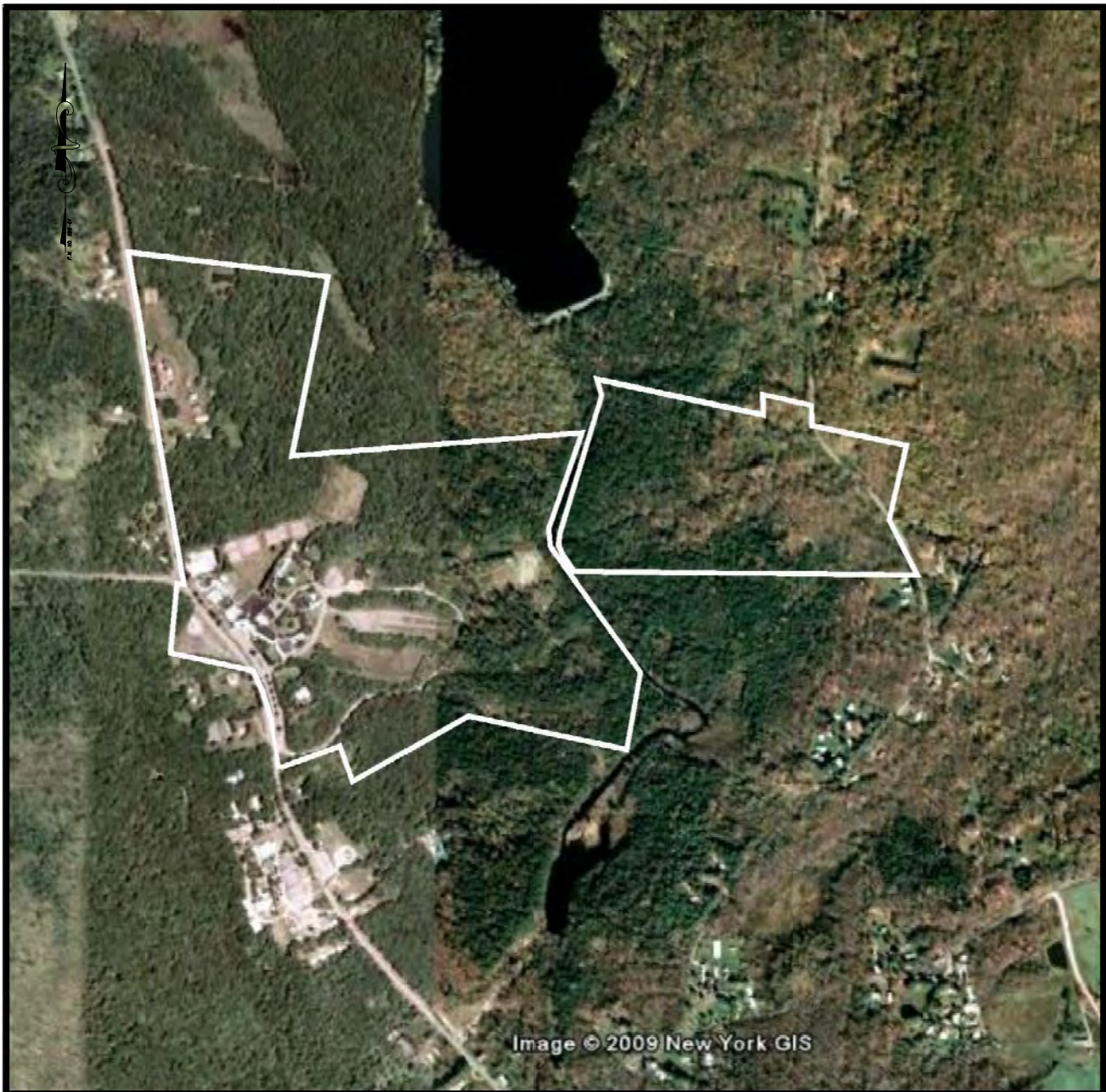
Figure 1: Aerial photograph of Raleigh Hotel site. (Source: Google Earth) Scale: Unknown.
