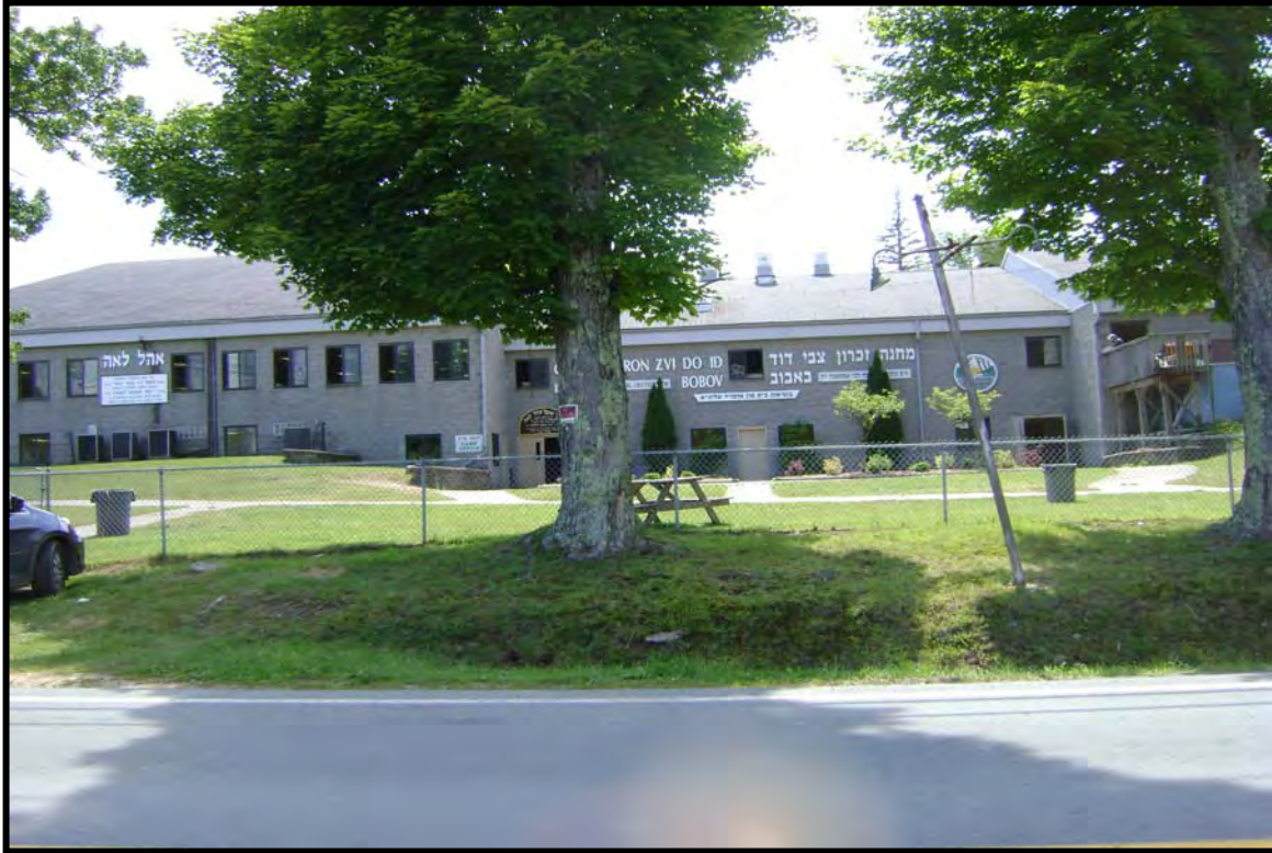
Photo 37: Yeshiva School located on western side of Heiden Road (CR 161) near Raleigh Hotel site. View west.
