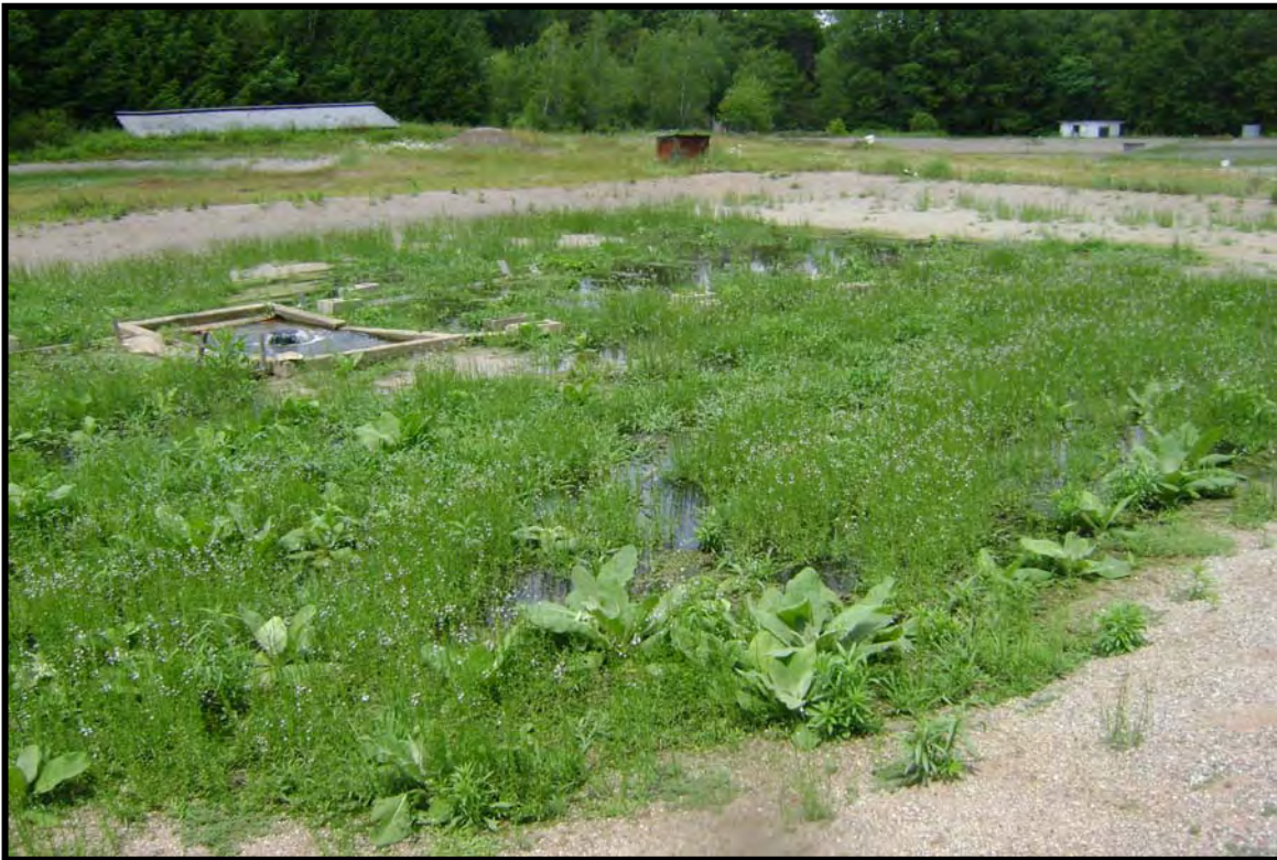
Photo 12: Sand filter bed with running water and pump or fountain in center. Area profoundly disturbed. View north.
