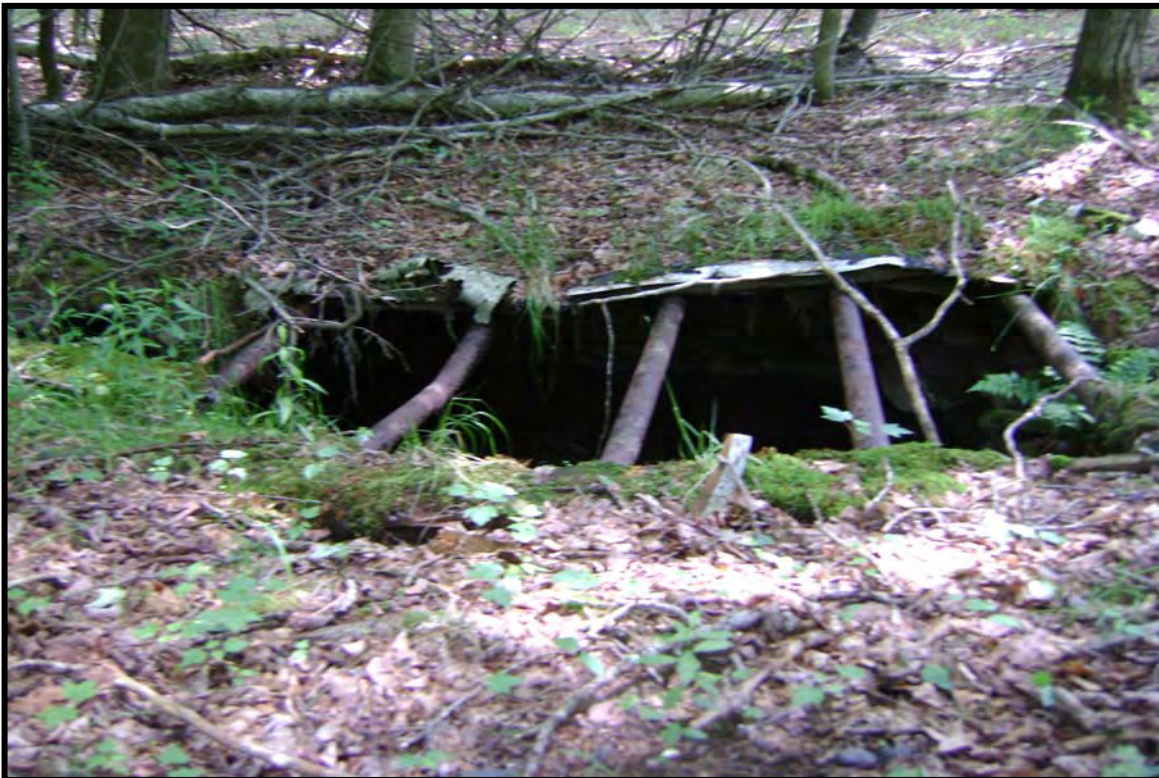
Photo 26: Oblong cistern, covered with bars and sheet metal located at start of Transect 114 along northern boundary of APE. View north.
