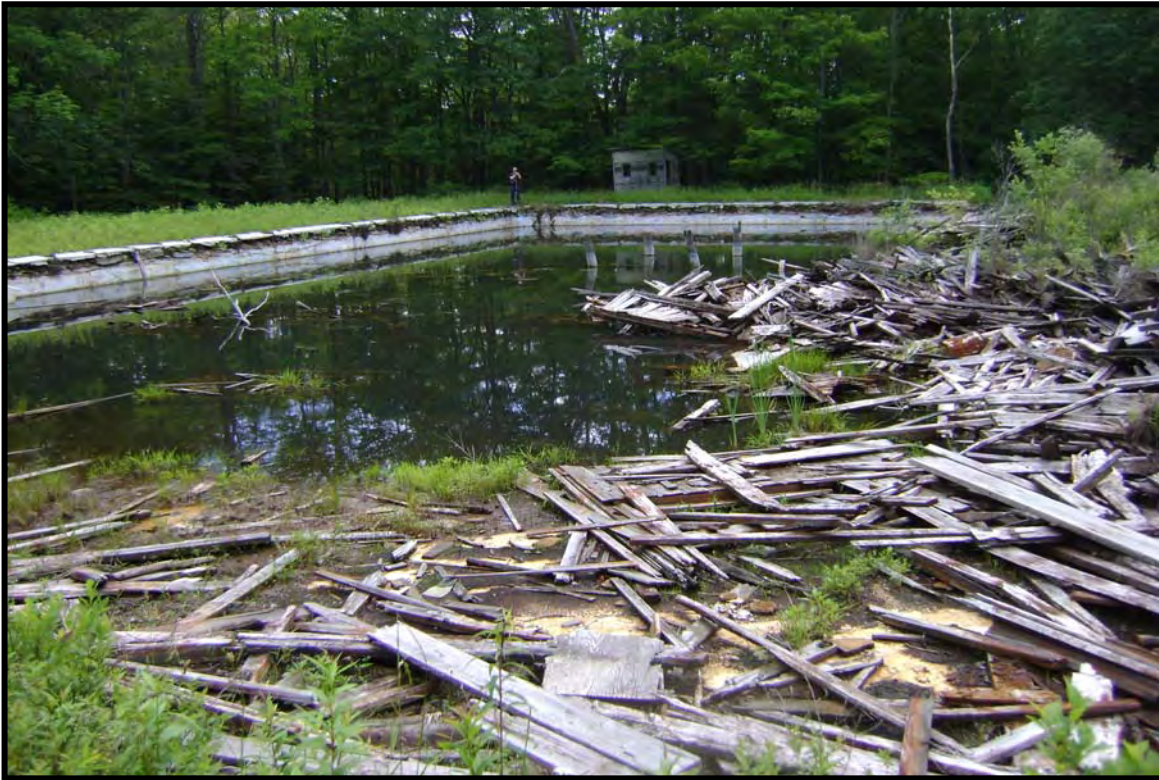
Photo 7: Large swimming pool in rear of Heiden Hotel parcel. View northwest.
