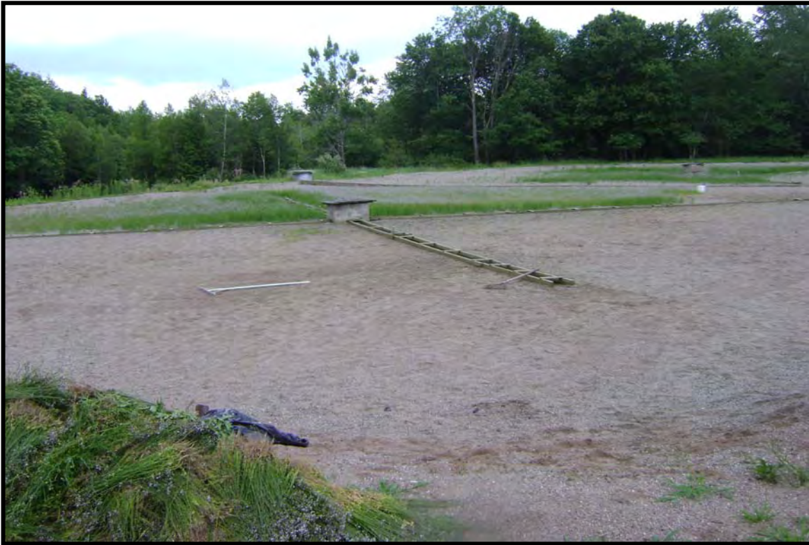
Photo 11: Sand filter beds are located within the central portion of the Raleigh Hotel Site. View to east.
