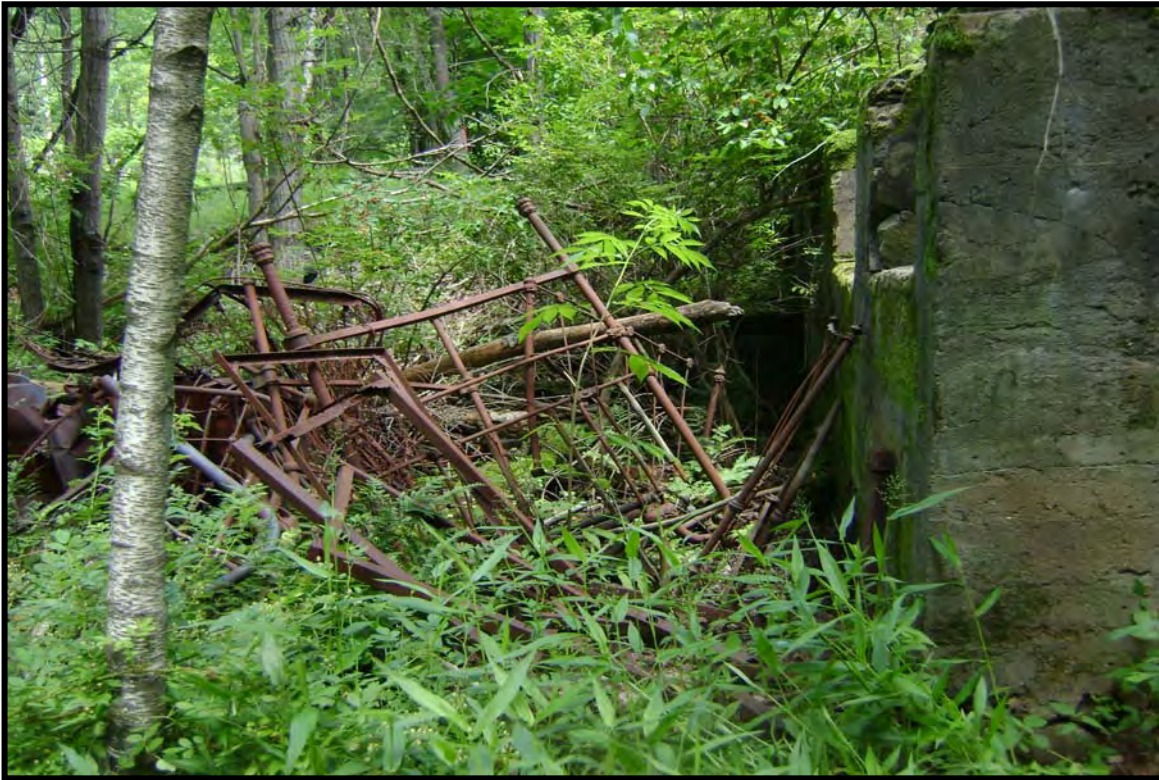
Photo 29: Interior of the foundation seen in Photo 28 is filled with metal, trash and debris. View north.
