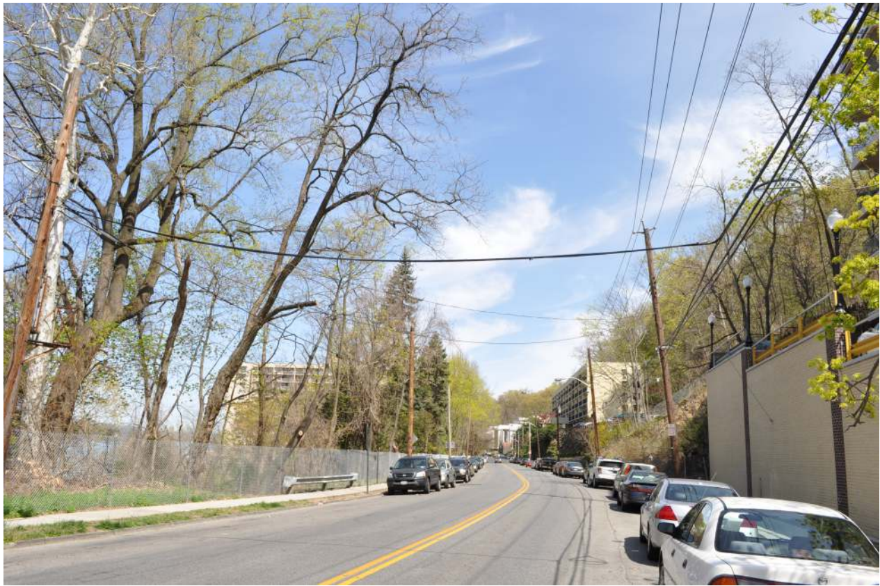
View 1N: Looking North - Project Site on Left
