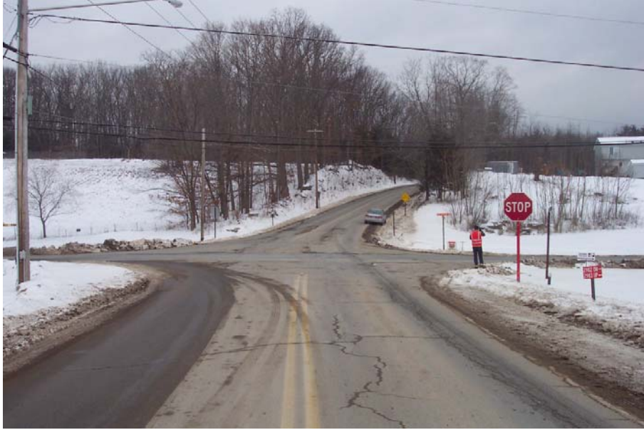
WESTBOUND BRUYN TURNPIKE APPROACH
