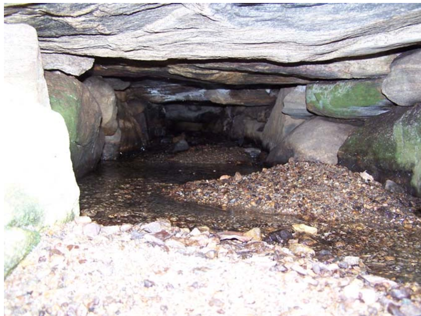
Photo 15: View southwest through stone culvert passing underground parallel to adjacent stream.
