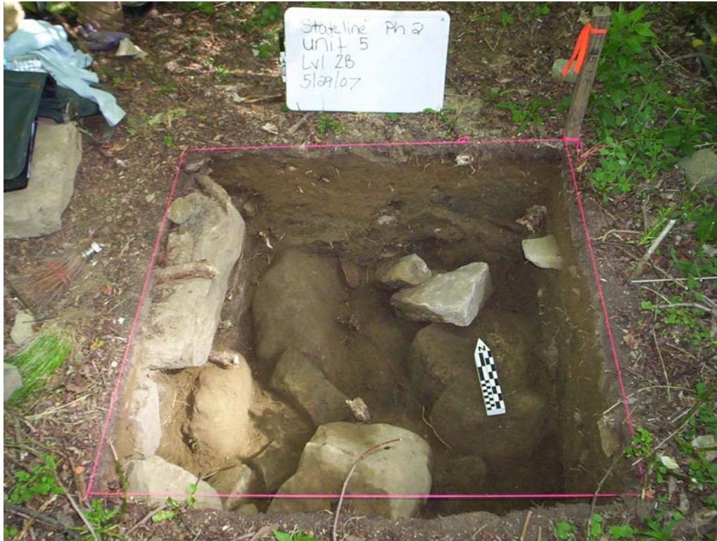
Photo 22: View north of Unit 5 during excavation. Foundation wall is along west wall at left.
