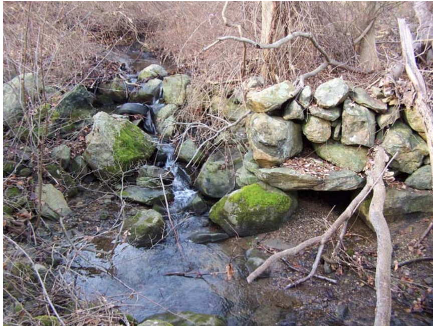
Photo 14: View southwest at stream cascade. Note dark cavity in stone work at right.
