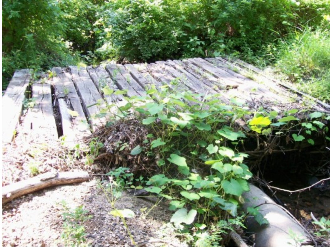
Photo 5: View west of bridge crossing stream.
