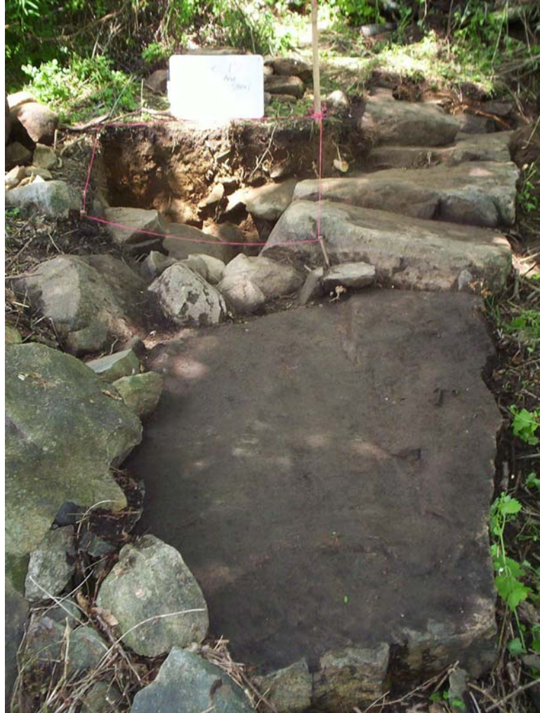
Photo 25: View north toward Unit 7 on the west side of foundation wall.
