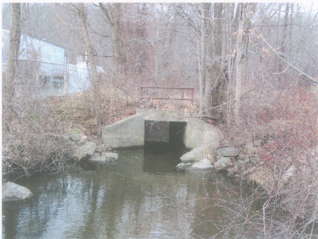
Photo 25: View north of old Route 6 bridge.
