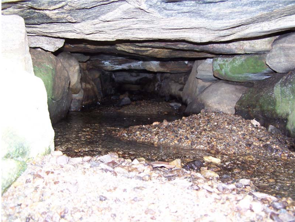
Photo 31: View southwest into stone culvert identified during Phase I investigation.
