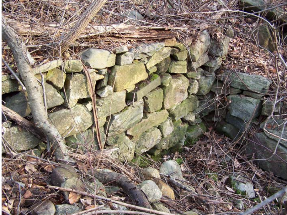
Photo 16: View northeast showing bridge foundation.
