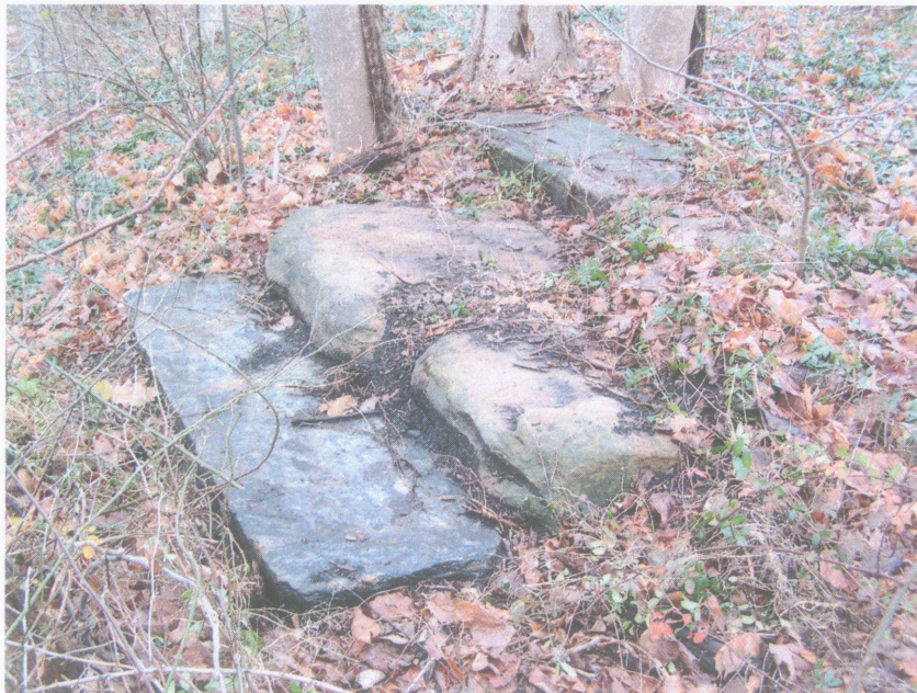
Photo 13: View northwest of School No. 1 steps and foundation on north side of U.S. Route 6 (outside of Project Area).
