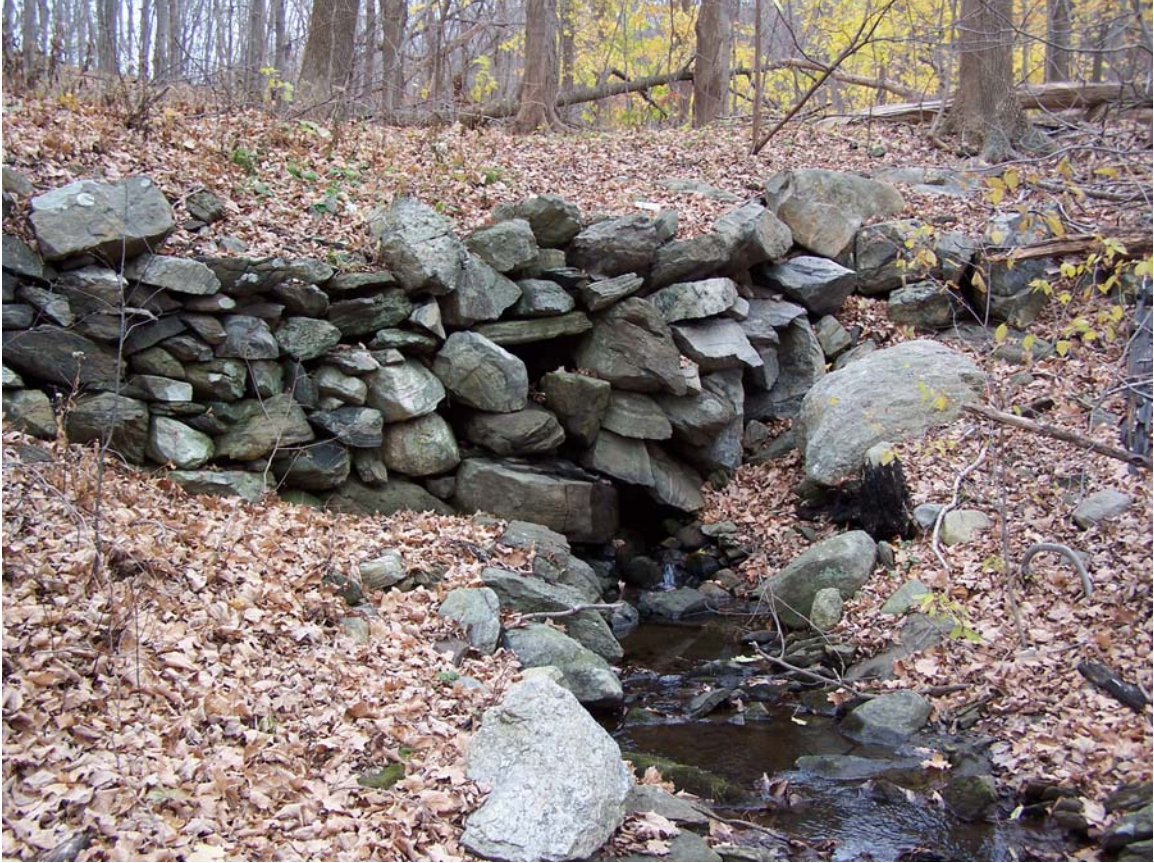
Photo 21: View south of stone culvert under old Route 6 in vicinity of historic D. F. Stevens residence.
