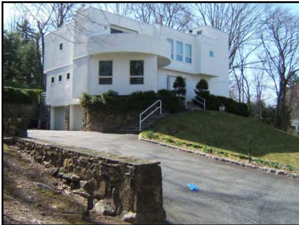
Photo 43: Modern house (47 New Street) is located on west side of New Street at entrance to project area. View to northeast.
