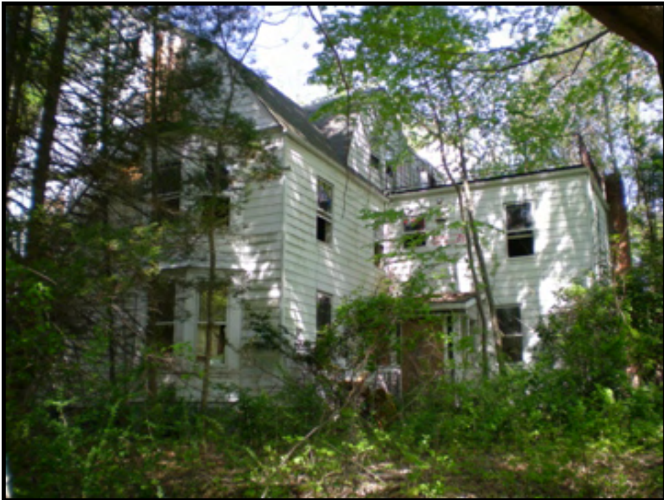
Photo 4: View of the southern side of Elliot House . View to northwest.
