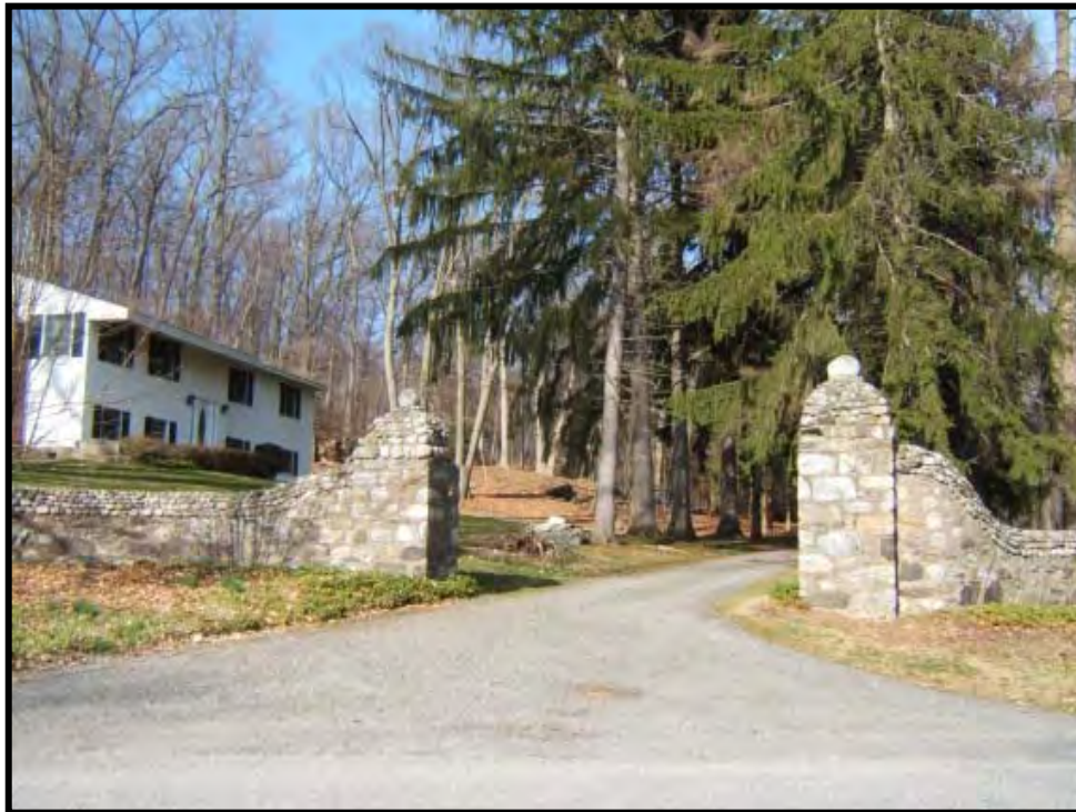
Photo 39: Stone gates flank drive that formerly crossed site to access New Street. Modern house to left is just outside project area. View to northeast.
