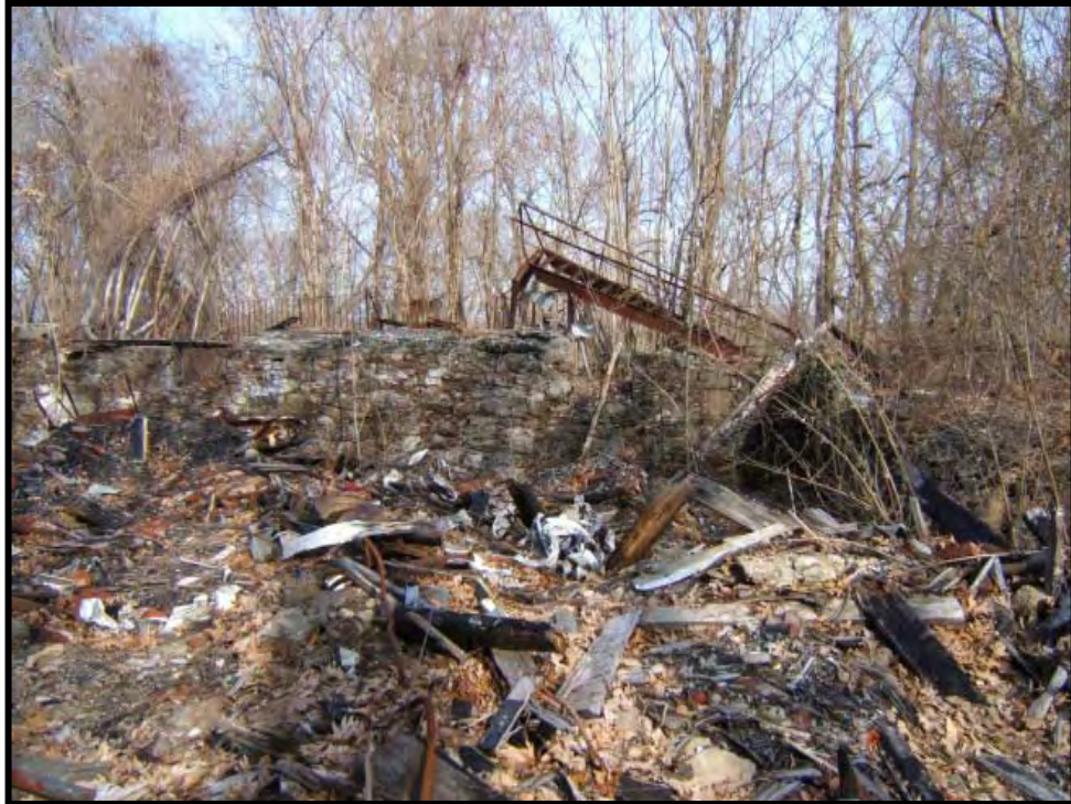
Photo 17: Looking south across cellar hole of Schmidt House . Note stairs for fire escape. View southeast.
