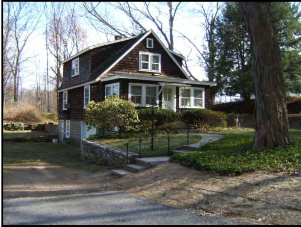
Photo 35: House located at 125 Harris Road is opposite southern boundary of project area dates to first half of 20 th century. View to south.
