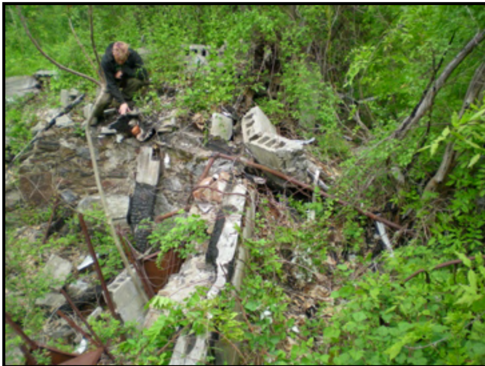
Photo 12: Schmidt House had parged fieldstone walls overlain by cinderblock and cement. View northeast.
