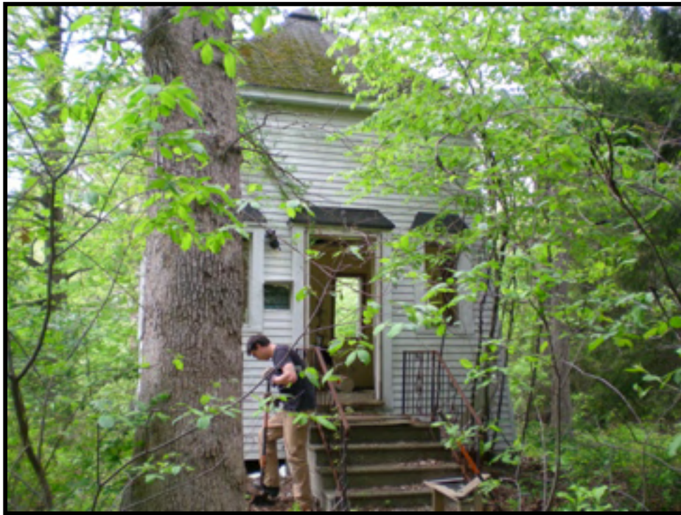
Photo 10: Field Crew testing perimeter of Cottage. View north.
