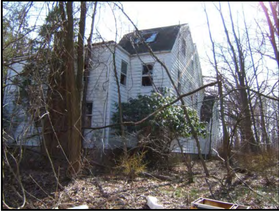
Photo 3: View of Elliott House northwest corner. Differing roof levels are indicative of additions constructed at different dates. Cartographic research indicates structure was built between 1914-1917. View southeast.
