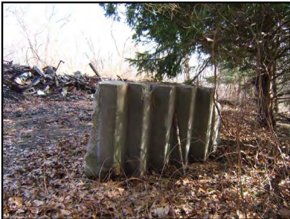
Photo 18: Concrete steps associated with rubble seen in background. Believed to have been an additional element of the Schmidt House. View to southeast.
