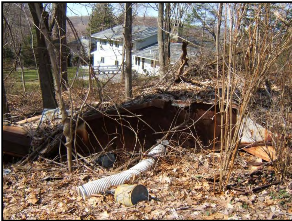
Photo 6: Collapsed metal shed on north side of house. House in background is located on Nightingale Road. Majority of houses around perimeter of project area were built in 20 th century. View to northeast.
