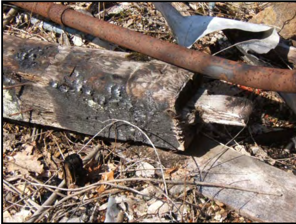
Photo 13: Mortise and tendon beam noted in debris pile at the “school” suggests construction date in late 18 th century or early 19 th century. It may be that some earlier material was used in construction of Schmidt House. View northwest.
