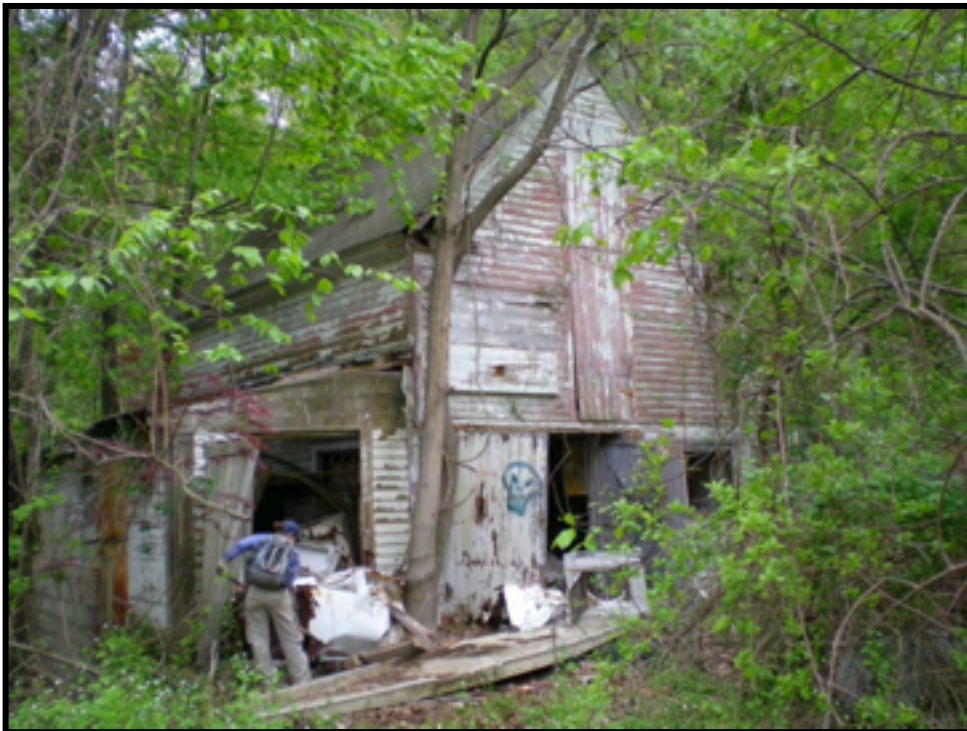
Photo 16: Two story garage associated with Bailey Hall. View west of field crew testing perimeter
