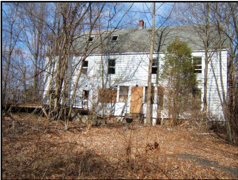
Photo 2: Elliott House located in northern portion of Tripi Subdivision site. House has been abandoned for some time, and is much deteriorated. View to northeast.
