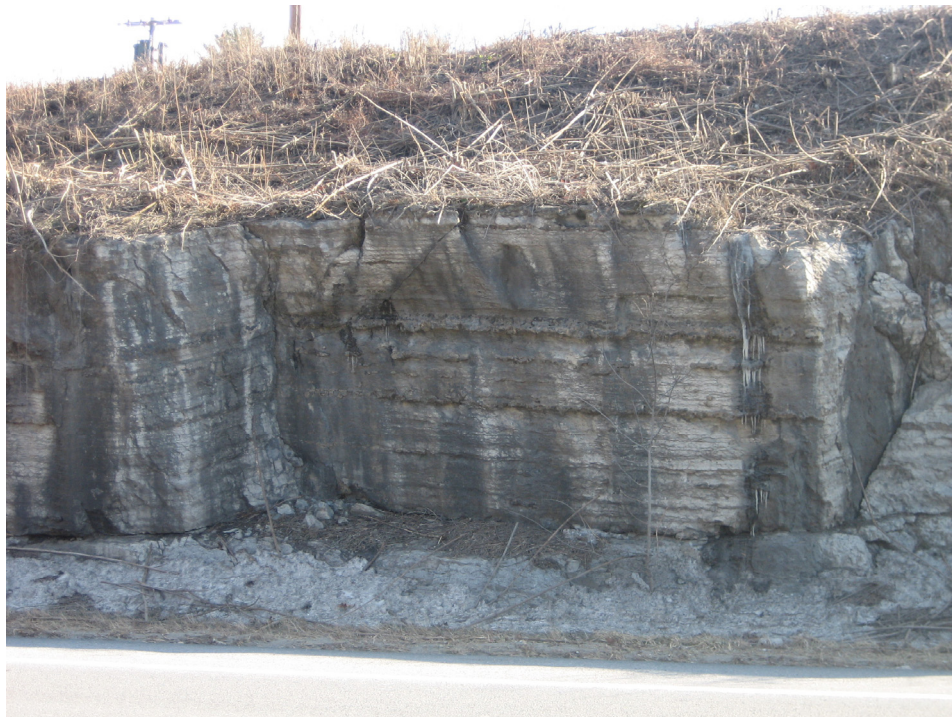
2) View of bedrock road-cut on Route 9W, directly west of site (facing east). Bedding and chert layers are visible. Solution is visible near rock surface.
