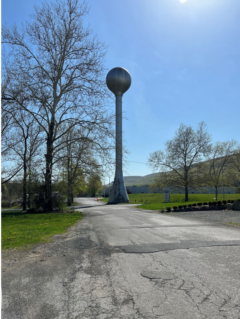
2) Existing Star Warehouse water tank (not in service), facing southwest.
