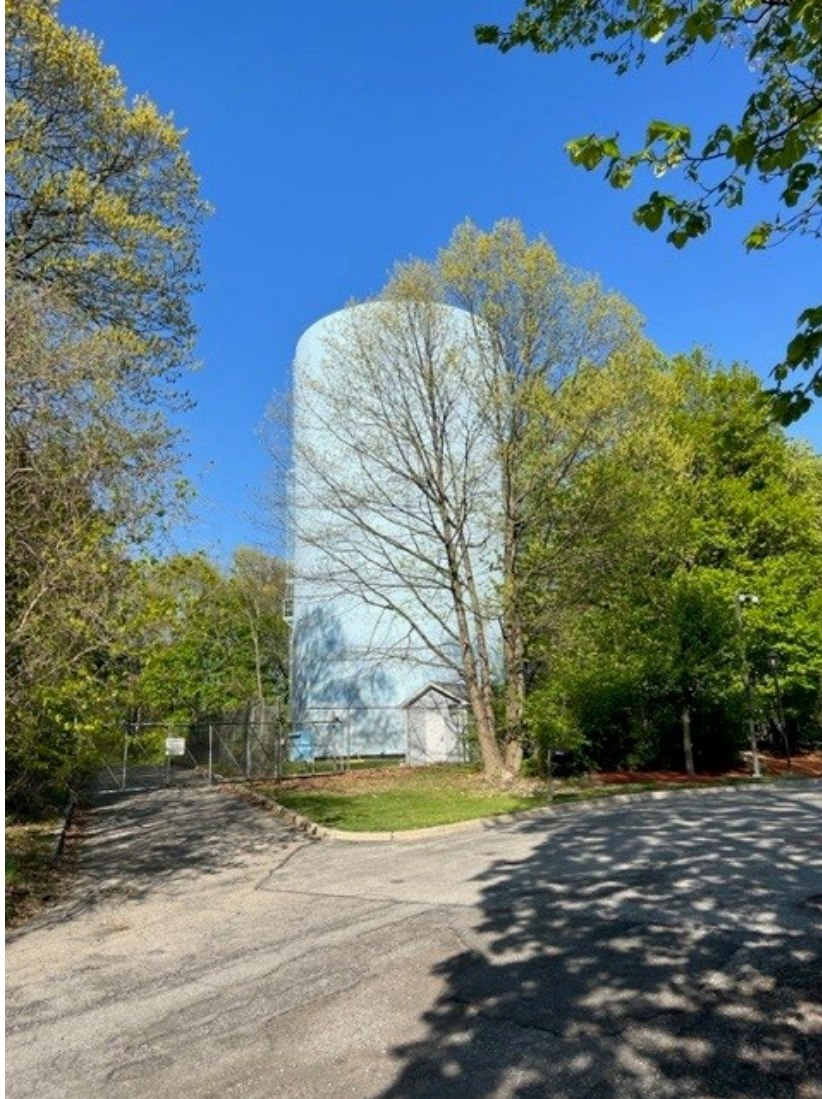
Figure 3.7-5 Existing Structures Photographs Star Warehouse Expansion, Town of Cornwall, NY
