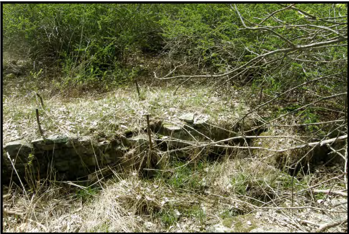
Photo 24: Stone remains are in location of MDS Tannery in Gilman's Station, outside project area. View south.
