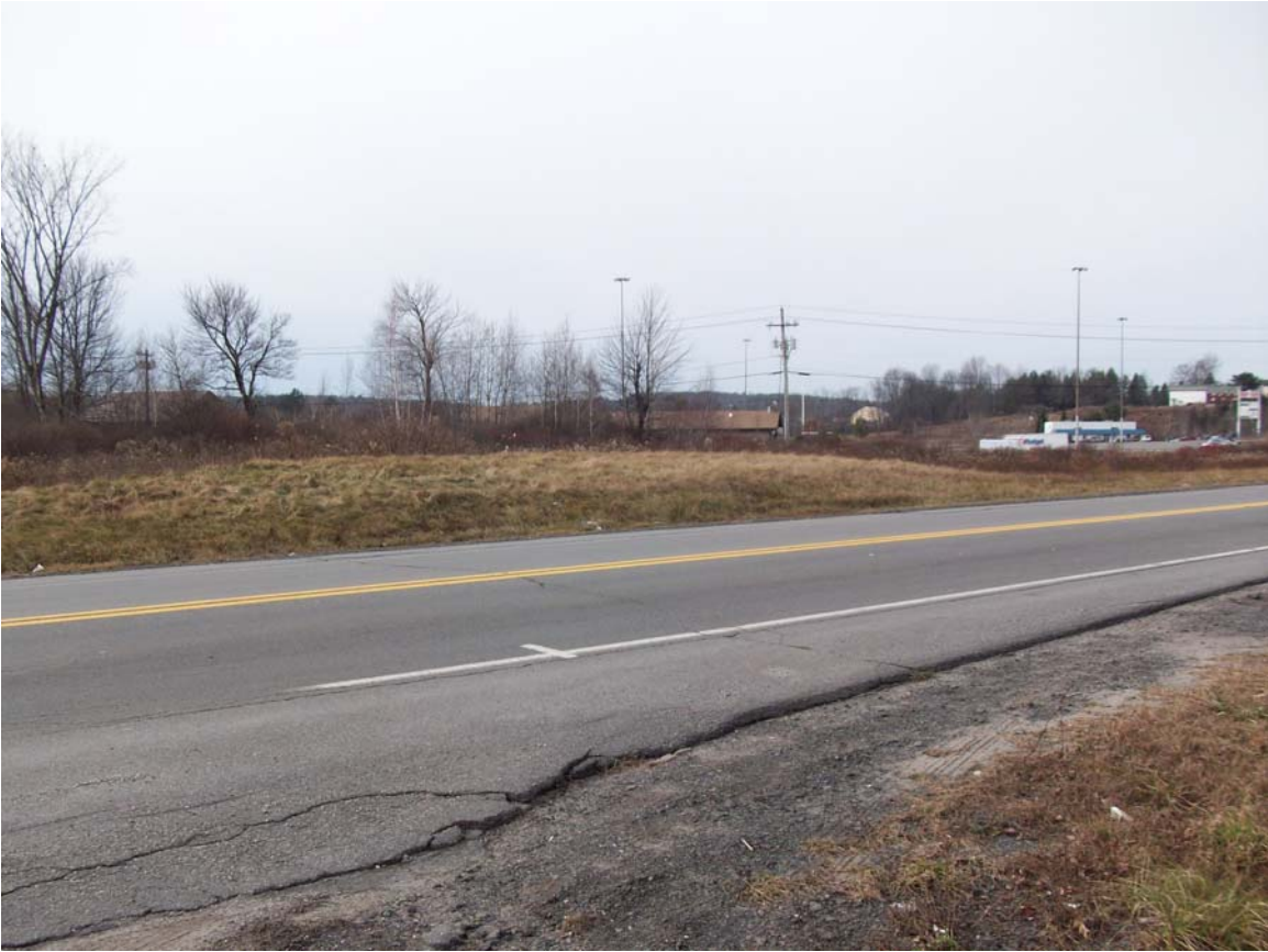
Photo 4C: Knoll on south side of CR 173 interfering with sight lines in Photo 4B Tim Miller Associates, Inc., Dec 2009.
