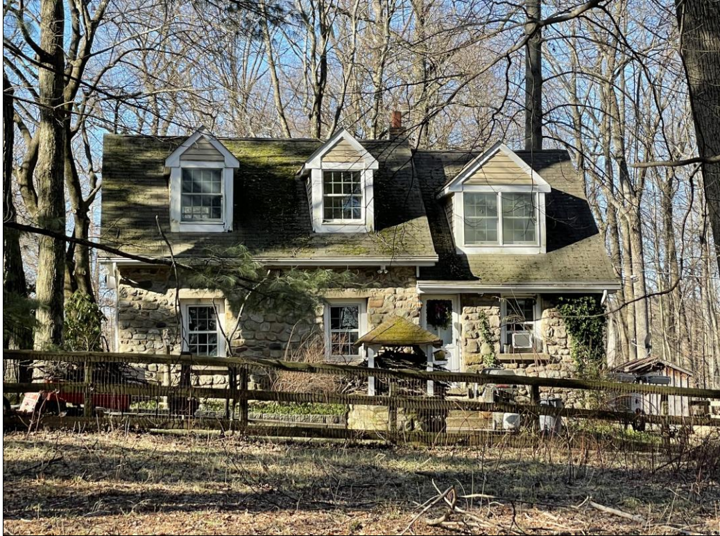
Photo 19: View west of Project Area showing front of house proposed for removal.
