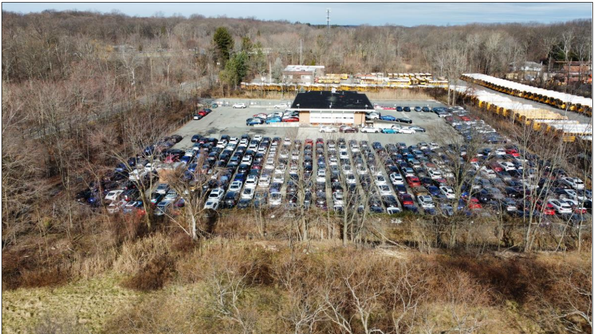
Photo 2: Aerial view north of Project Area showing Con-Way Freight yard proposed for redevelopment.
