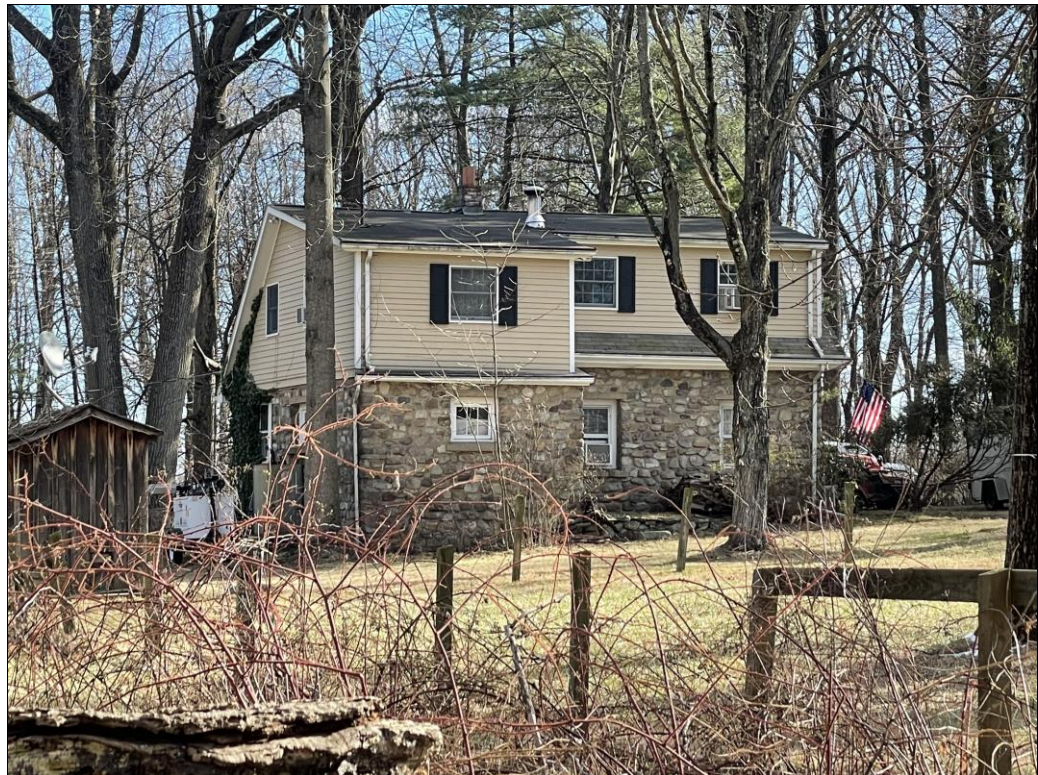
Photo 20: View southeast of Project Area showing rear of house proposed for removal.
