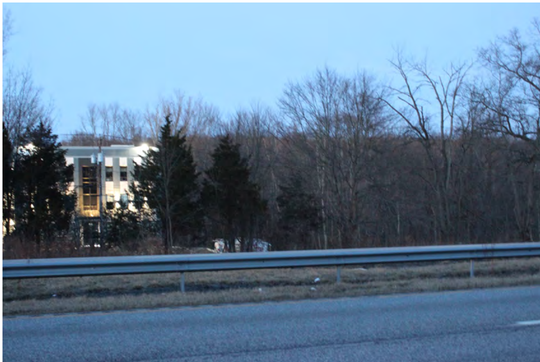
4) Location 5 View of project site from NY Route 17 eastbound, facing northeast (Dusk condition)
