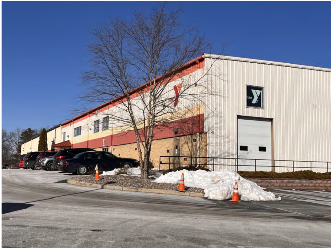
16) View of adjacent Southern Orange YMCA building, facing northeast.
