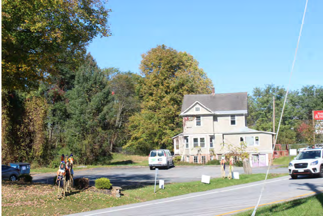
5) Location 3 – View towards project site from Schynnemunk Street and Route 208, facing northwest. Site includes former bicycle shop in photo.
