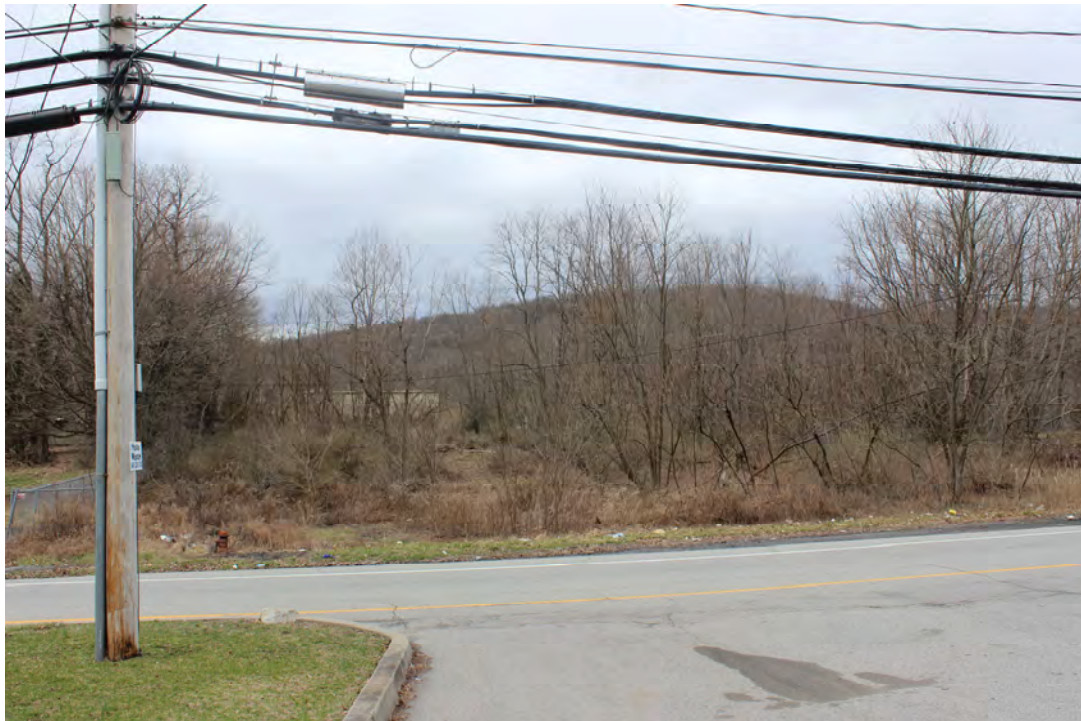
2) Location 1 - View of subject Property frontage on Route 208, with proposed site entrance, facing west. YMCA building is in background.
