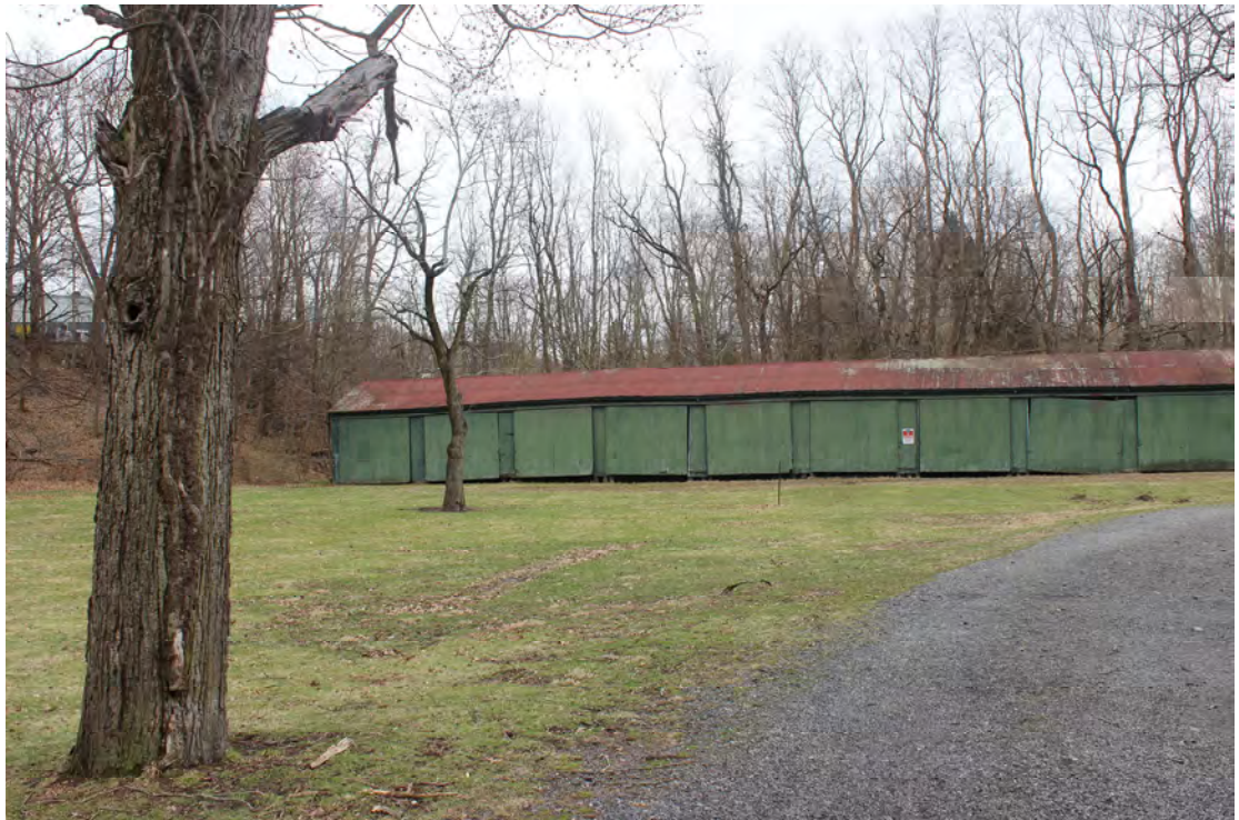
12) Location 6a - View of Property in winter months, facing southeast.
