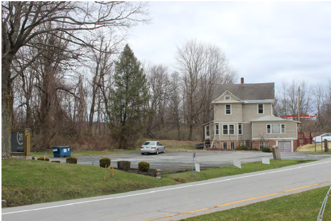
6) Location 3 - View of subject Property in winter months, facing northwest. Exxon station is at right.
